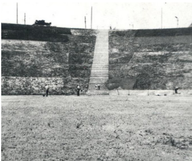
Figure 26. The stone steps and amphitheatre at Cooper Park during construction in the 1930s (source: Woollahra Libraries)
