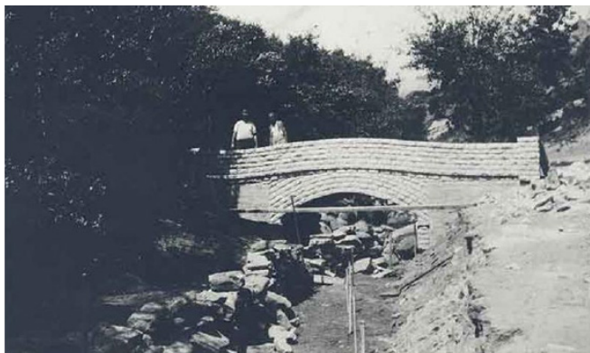
Figure 25. Two workers on the Moon Bridge during construction in the 1930s (source: Woollahra Libraries)
