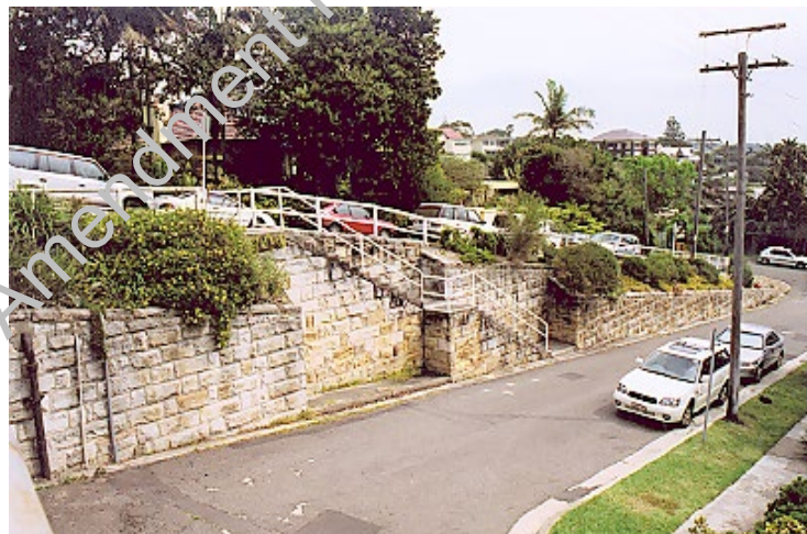
Sandstone retaining wall along Salisbury Street
