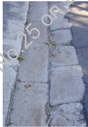
Sandstone guttering
