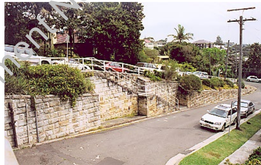
FIGURE 91 Significant sandstone retaining wall
