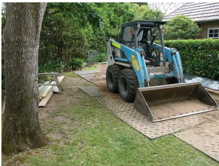
Figure 4 – Showing typical detail for truck mats.
