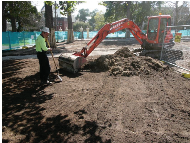
Figure 5 – Showing method for removal of residual surface vegetation from Tree Protection Zones following herbicide treatment and slashing.
