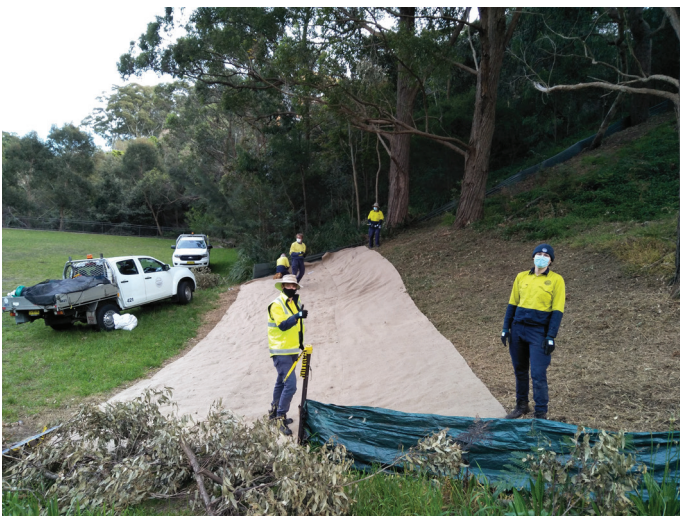
Planting works at Cooper Park
