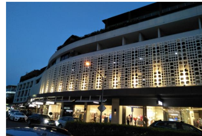
Up lighting of the Cosmopolitan Building
