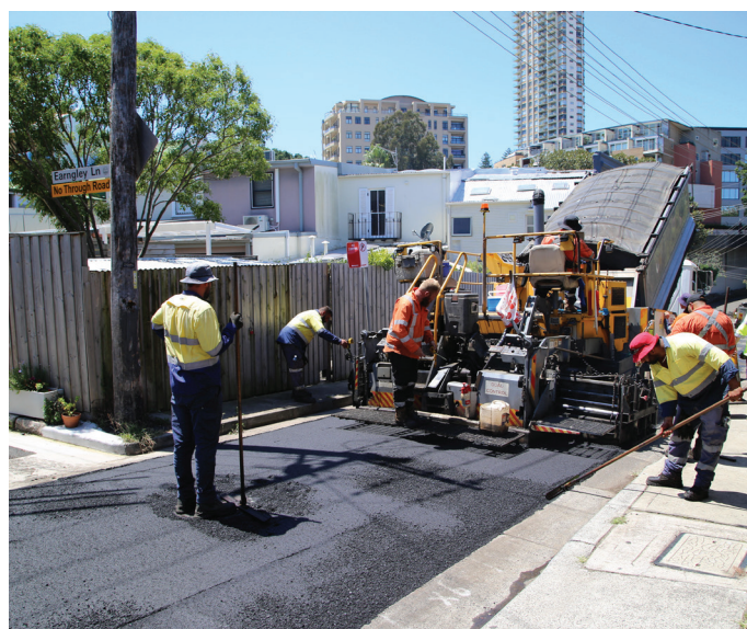
Road re-surfacing works in Edgecliff
