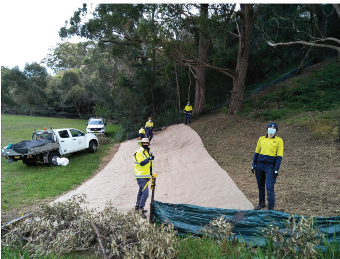
Planting works at Cooper Park
