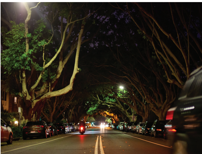
LED streetlights in Rose Bay
