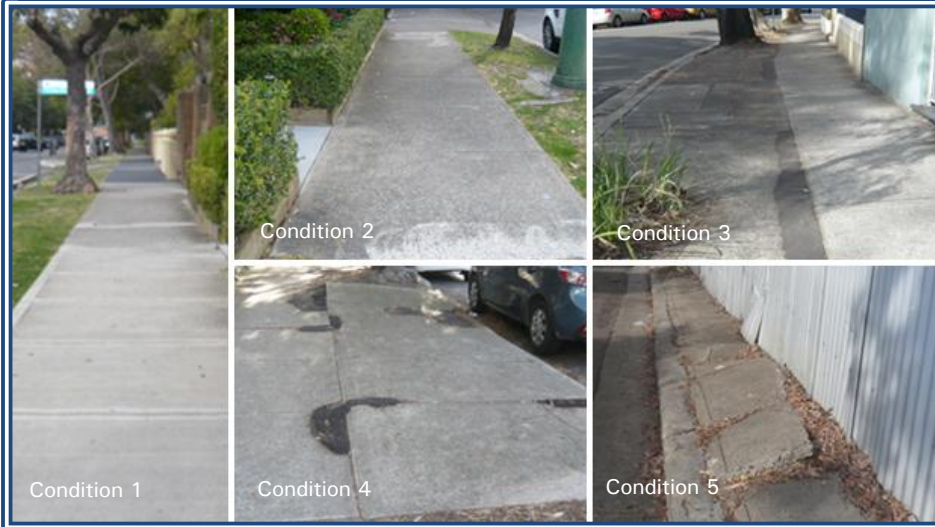
Example of condition ratings: Concrete footpaths
