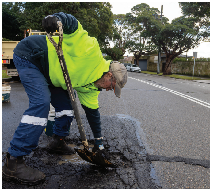
Pothole repairs after heavy rain event
