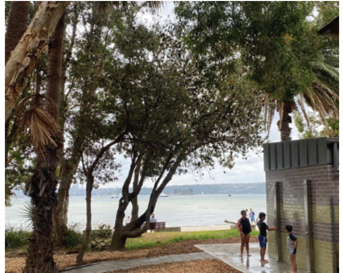
New amenities block in Percival Park, Rose Bay opened 23 December 2021
