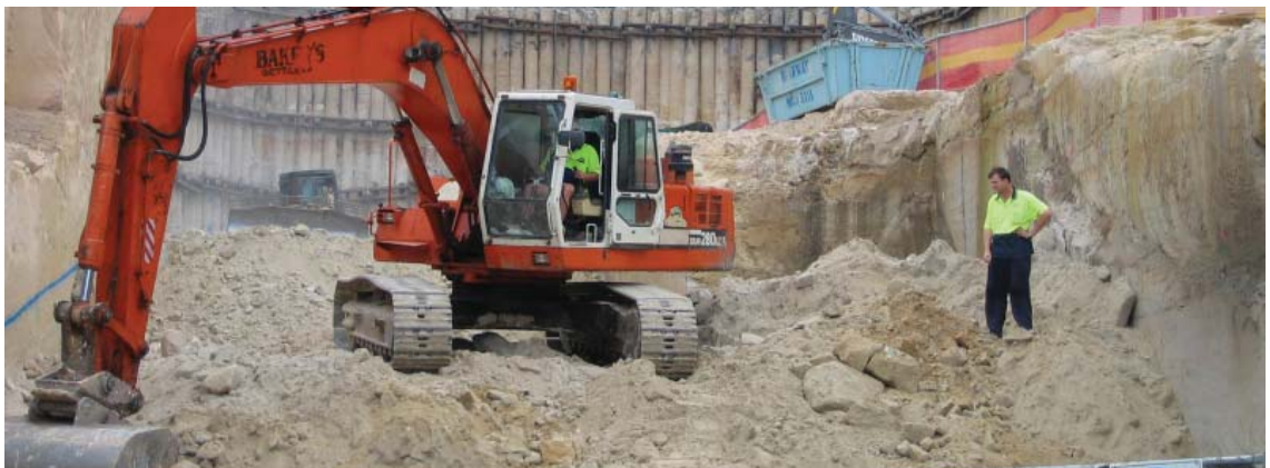
Photo: Woollahra Municipal Council
