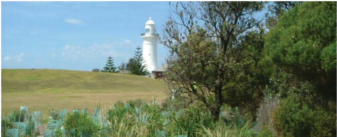
Photo: Woollahra Municipal Council
