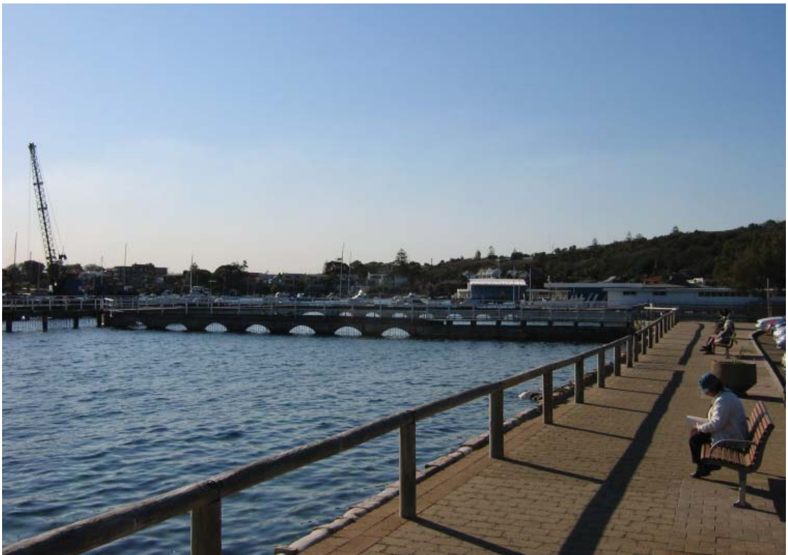
Photo: Woollahra Municipal Council
