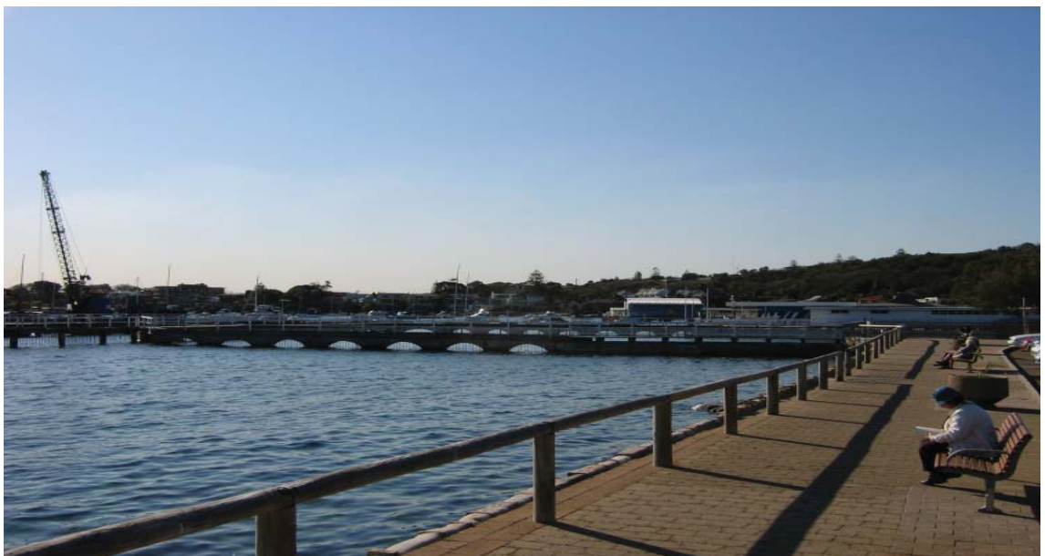
Photo: Woollahra Municipal Council
