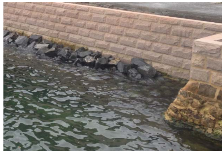
A small section of the new Lyne Park seawall
