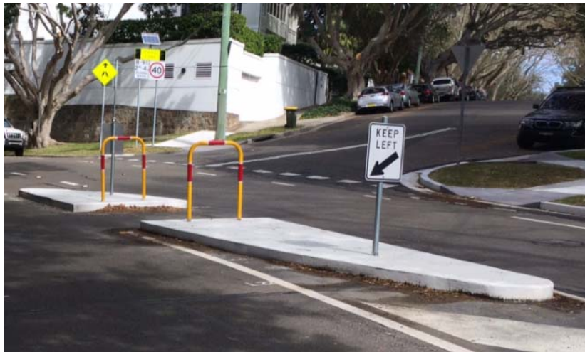
Pedestrian Refuge – Edgecliff Road at Wellington Street
