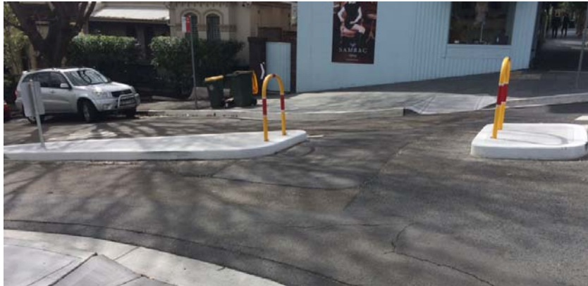
Pedestrian Refuge – Bathurst Street at Edgecliff Road
