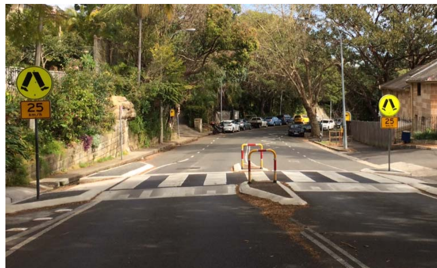
Pedestrian Crossing – Victoria Road, Bellevue Hill
