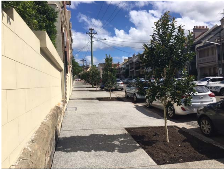
Suffolk Street footpath works
