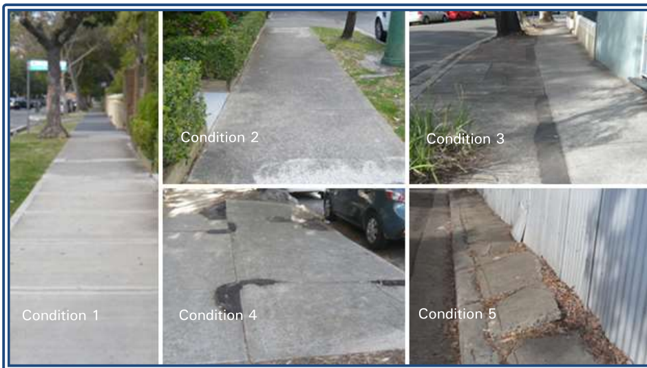
Example of condition ratings: Concrete footpaths
