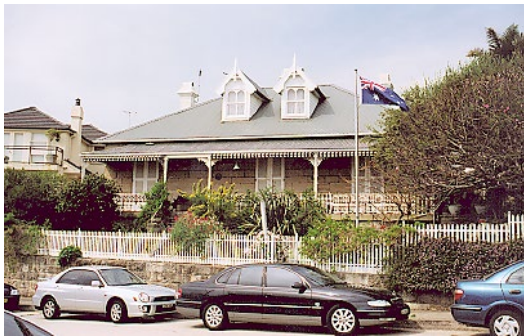
FIGURE 90 Contributory item on east side of Hopetoun Avenue
