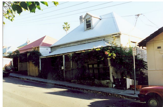
Timber weatherboard cottages in Cliff Street
