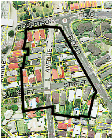
FIGURE 88 Aerial of the precinct
