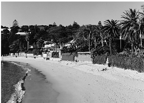
FIGURE 58 Camp Cove Beach frontage
