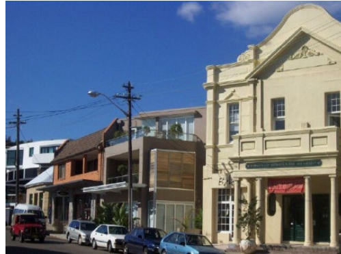
FIGURE 25 East side of Military Road, north of the Town Hall
