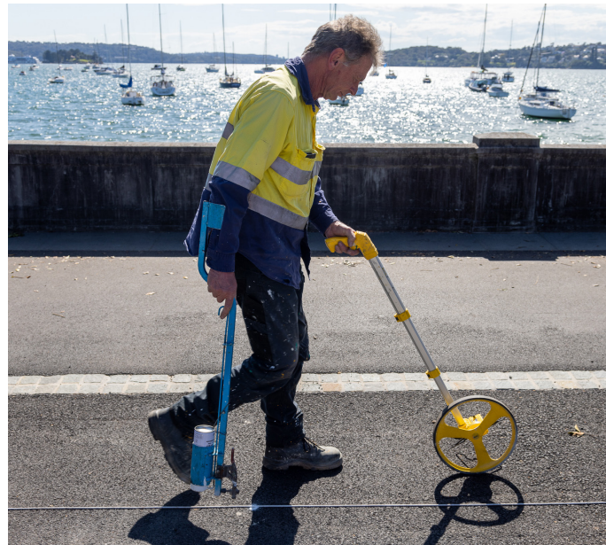
Rose Bay promenade cycleway line marking preparations
