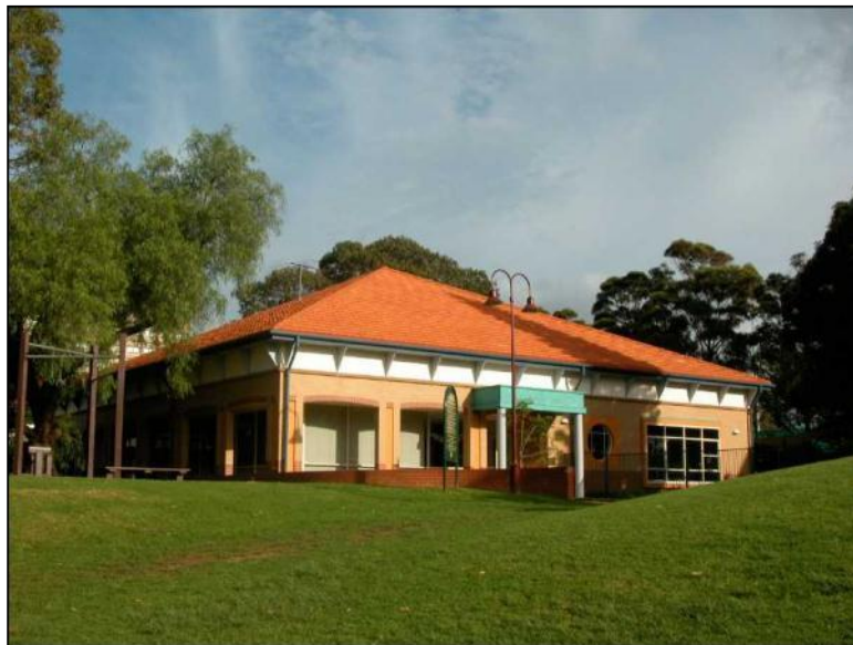
Figure 17: North Sydney Community Centre
