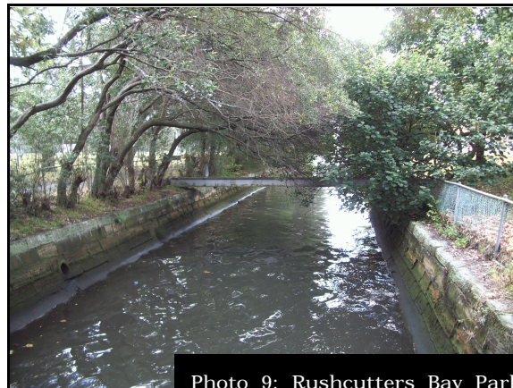
Photo 9: Rushcutters Bay Park, looking d/s
