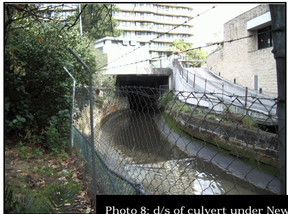
Photo 8: d/s of culvert under New South Head Road
