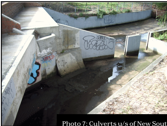
Photo 7: Culverts u/s of New South Head Road
