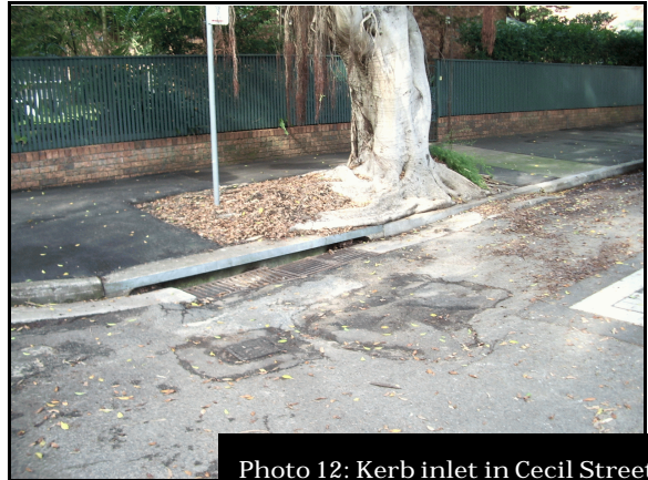
Photo 12: Kerb inlet in Cecil Street
