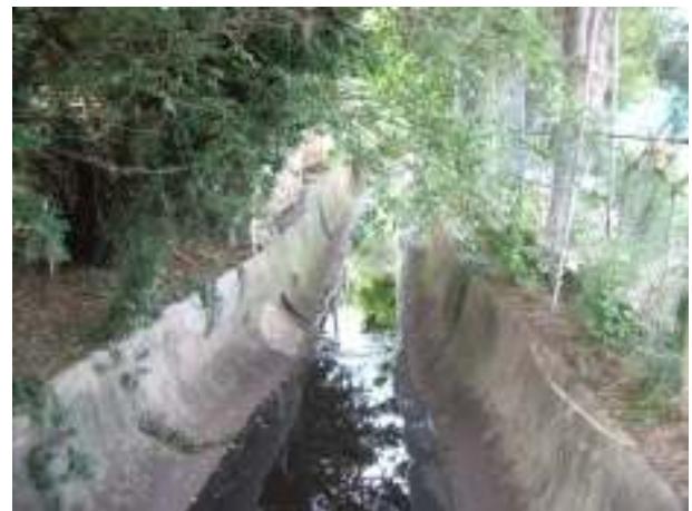
Photo 2 Looking u/s from footbridge within White City tennis complex
