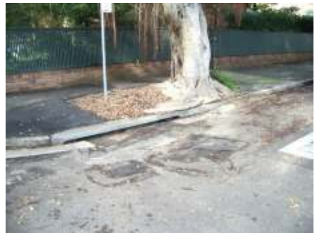
Photo 12 Kerb inlet in Cecil Street
