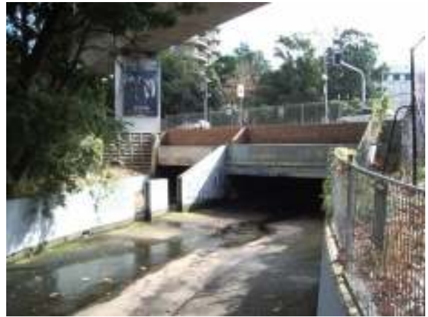
Photo 6 u/s of New South Head Road culverts
