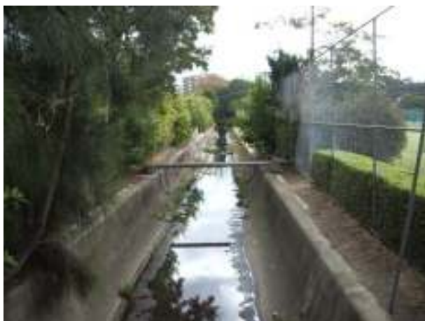
Photo 3 Looking d/s from footbridge within White City tennis complex
