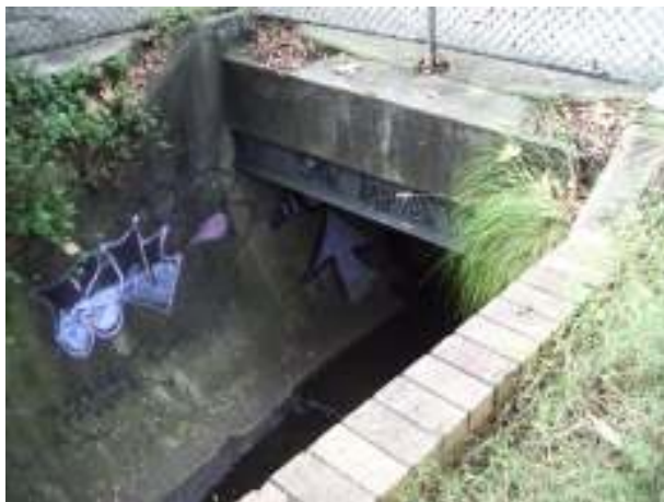
Photo 1 Open Channel d/s of Glenmore Road
