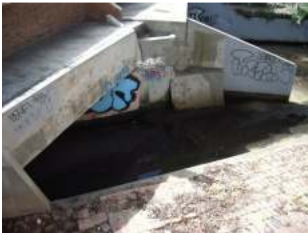
Photo 7 Culverts u/s of New South Head Road
