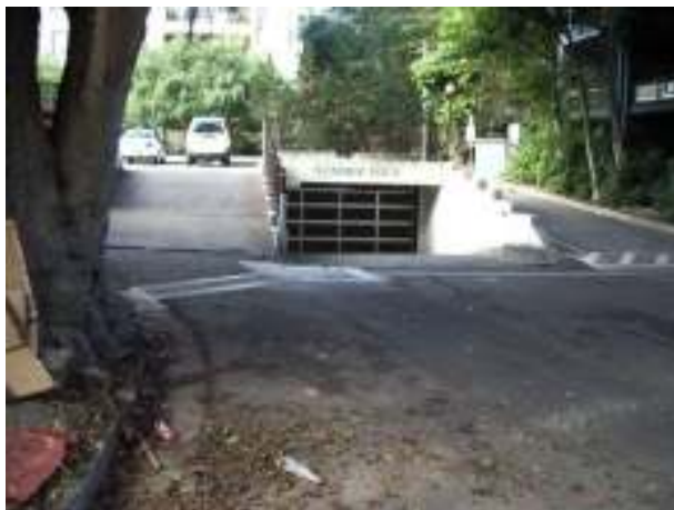
Photo 11 Grate inlet in front of underground car park, Hampden Street
