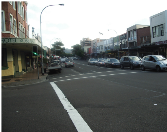
Photo 5: New South Head Road at Rose Bay looking west
