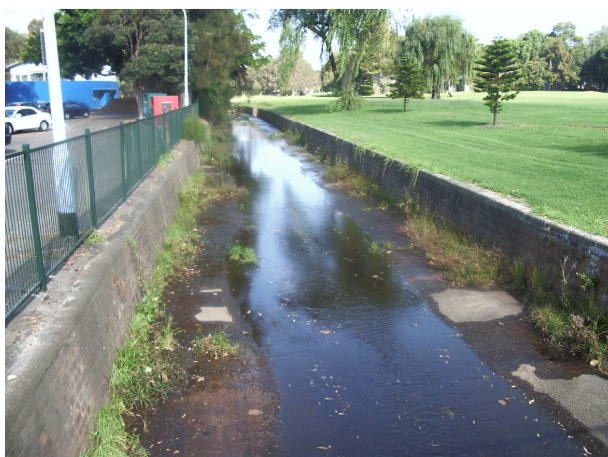
Photo 1: Open channel at Manion Avenue looking upstream
