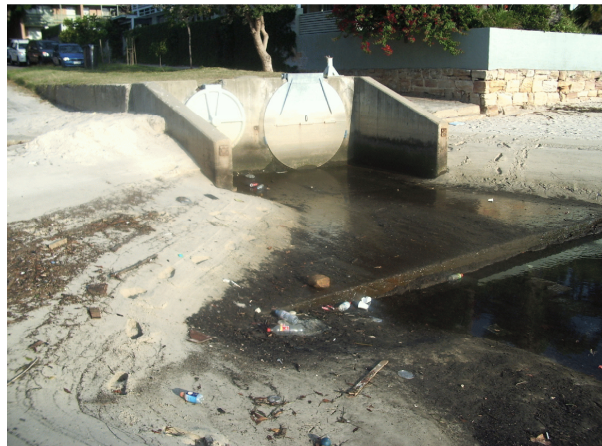
Photo 8: Stormwater outlet at the end of Caledonia Road
