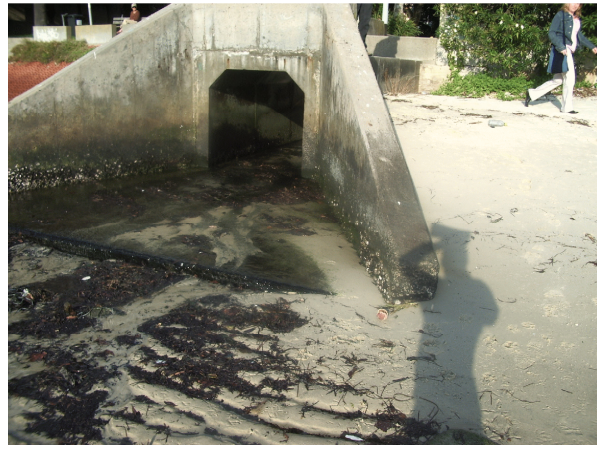
Photo 4: Storm water outlet at Rose Bay
