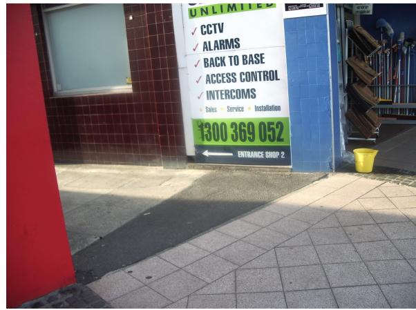
Photo 6: Worth Arcade which provides the drainage outlet to Rose Bay
