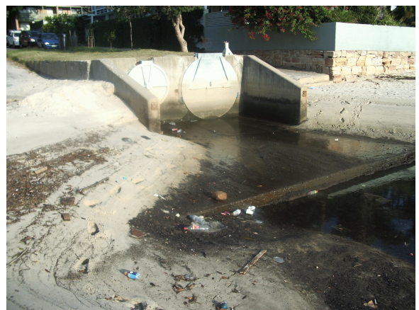
Photo 10: Stormwater outlet at end of Caledonia Road
