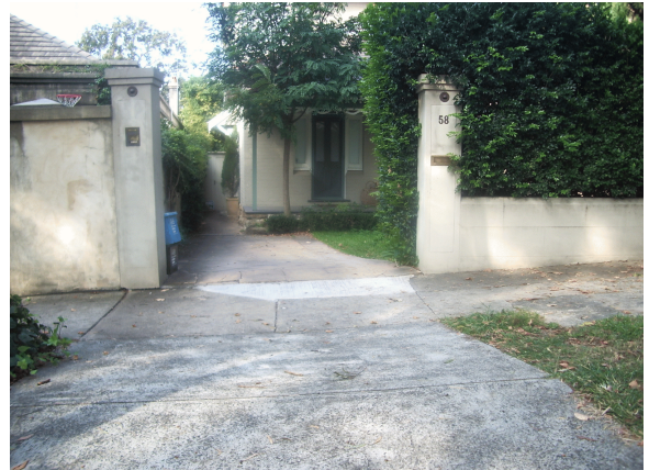
Photo 4: Footpath and carport below level of road at Latimer Road
