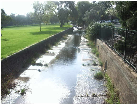
Photo 3: Open channel at Manion Avenue looking downstream
