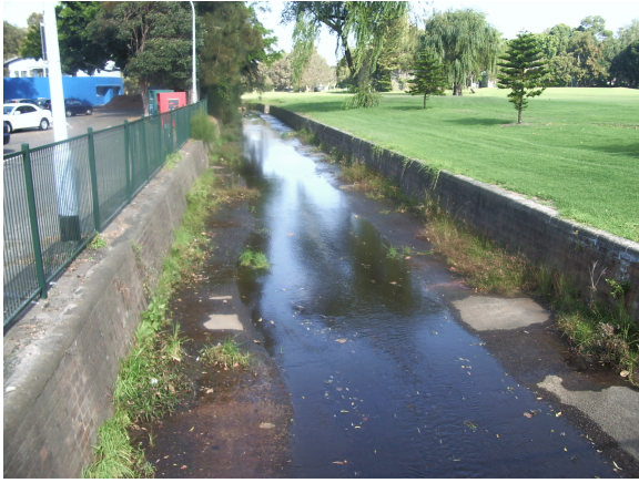
Photo 1: Open channel at Manion Avenue looking upstream
