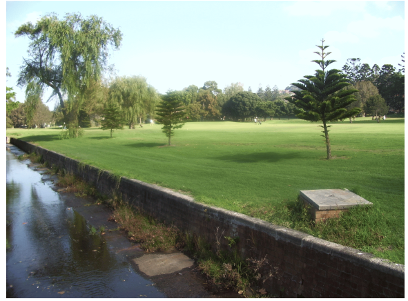
Photo 2: Open channel at Manion Avenue looking upstream
