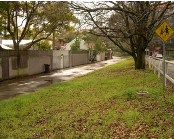
Photograph No. 3. Covered channel next to Sherbrooke Avenue, looking towards harbour.
