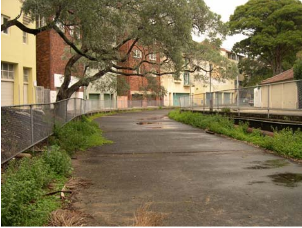
Photograph No. 2. Covered channel between Jamberoo Lane and Cross Lane, looking towards New South Head Road.
