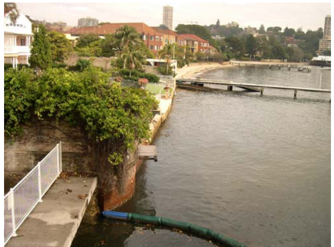
Photograph No.4. View of harbour foreshore with main stormwater outlet in foreground.
