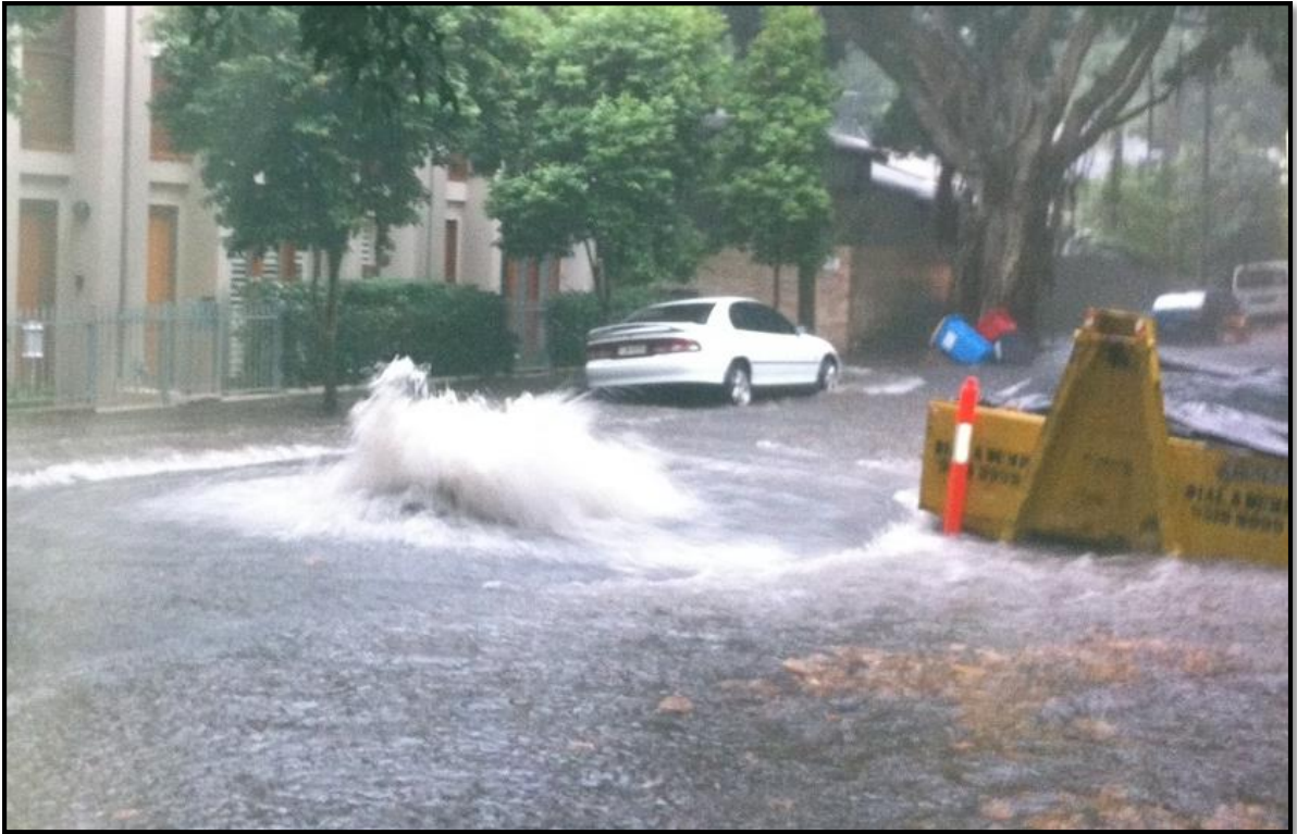
Plate 3 Surcharging stormwater pit in Hampden Street during April 2012 flood
