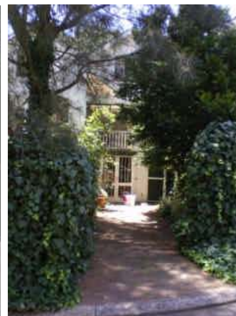
23. Ground floor Inundation Example of property at risk at Sutherland Ave
