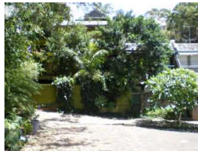
35. Ground Floor Inundation or Floor Below Road Properties with above floor level inundation recorded. Most likely flow from rear end where Sutherland Ave lies above floor level.
