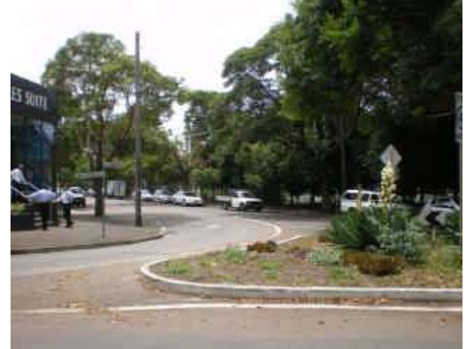
72. Ponding Intersection Boundary St\Nield Ave
