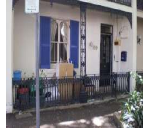
159 Paddington St Ground seepage enters residence during storms.
