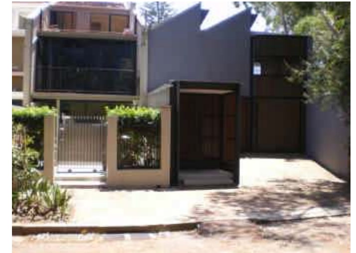
108. Ground Floor Inundation Example of properties on Cecil St at risk of inundation.
