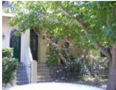
133 Windsor St Above floor flooding due to local drainage problem
