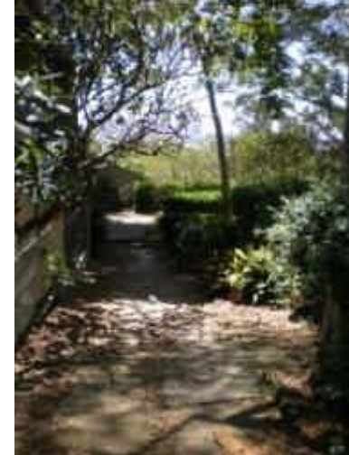
30. Flow Diversion Possible flowpath to lower Harris Street
