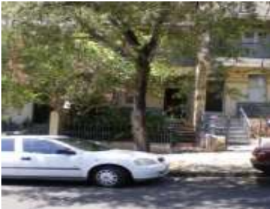
311 Glenmore Rd Groundwater seepage due to storm events.
