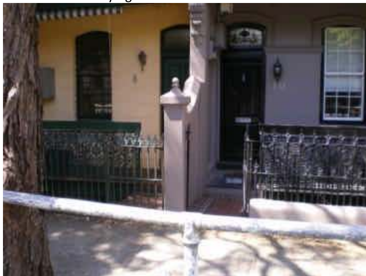
41. Floor Below Road Low point in Hargrave St. Inundation of lower levels likely for several properties
