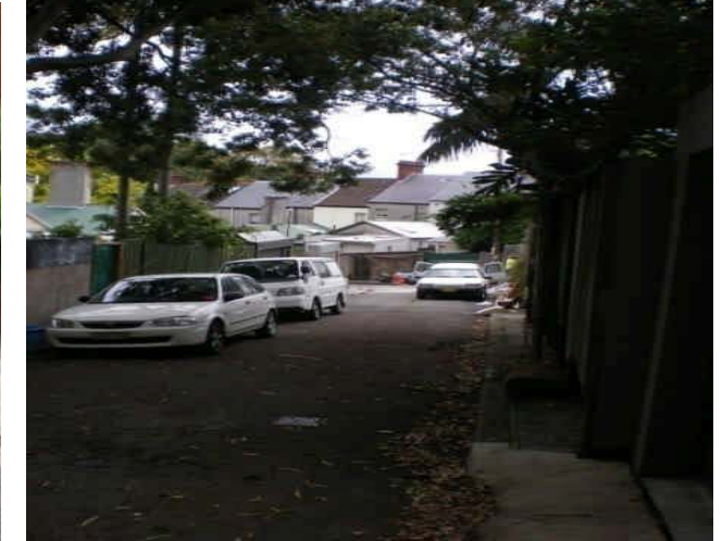
68. Flow Diversion Possible flow path from Liverpool St through Boundary Ln to Boundary Street
