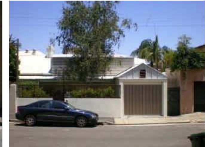
16. Flow Diversion Previously inundated above floor level, but fence and garage now in place to divert flow
