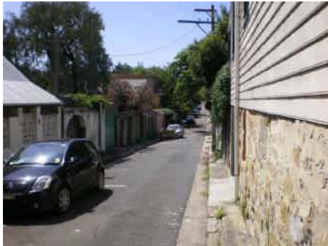
85. Ponding Hargrave Ln low point.
