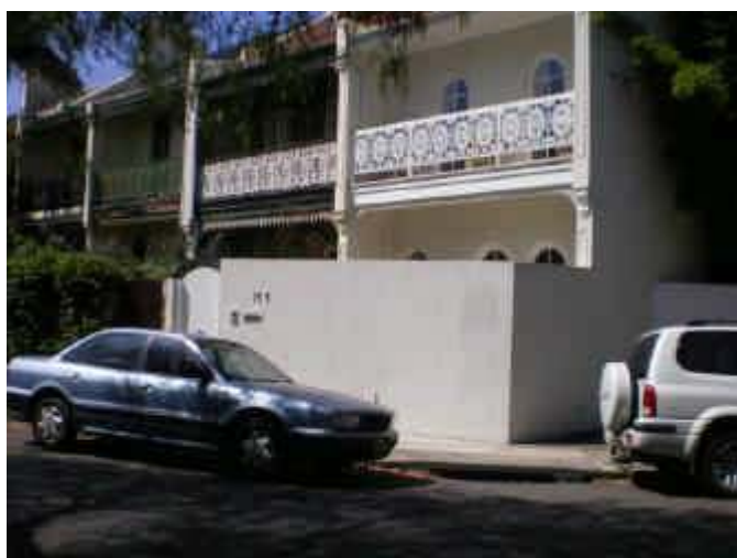
57. Flow Diversion Previous reports state water reached a level 0.15 m below the floor at No. 21. The protective walls at both No 21 and 19 could increase problems at adjacent properties.
