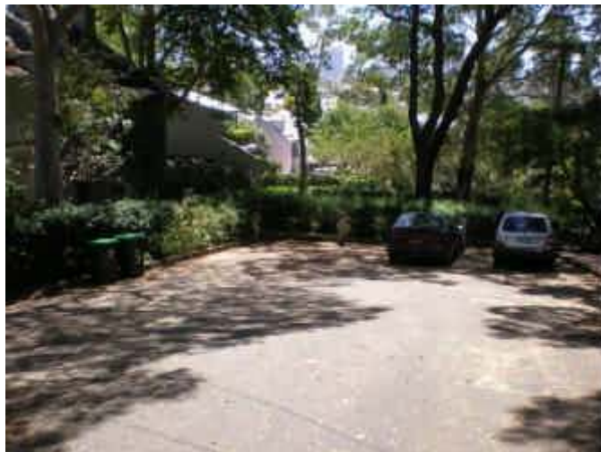
29. Ponding & Flow Diversion Upper part of Harris Street. Possible flow path (see 30) to left in picture
