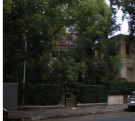
113 Jersey Rd Major overland flows and severe flooding during stated events (1984, Jan 87, Jan 89, Apr 89, and Jan 91). (blamed on regrading of park in 1987, barricades now exist diverting flow and have prevented above floor flooding).
