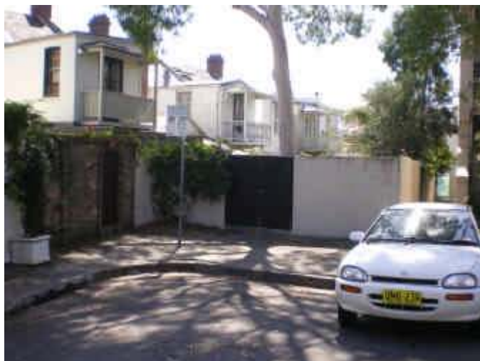
117. Ponding & Ground Floor Inundation Ponding at the end of Hopetoun St
