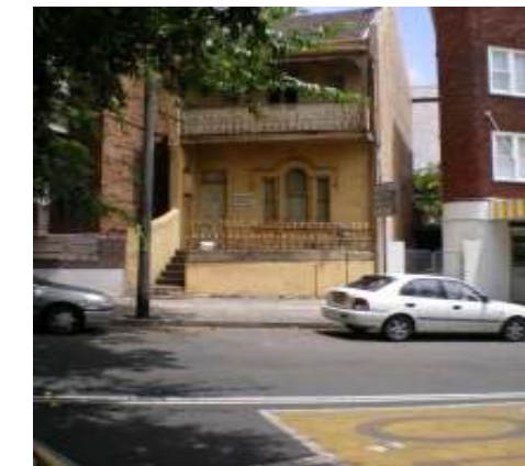
1 Gurner St Groundwater seepage due to storm events.
