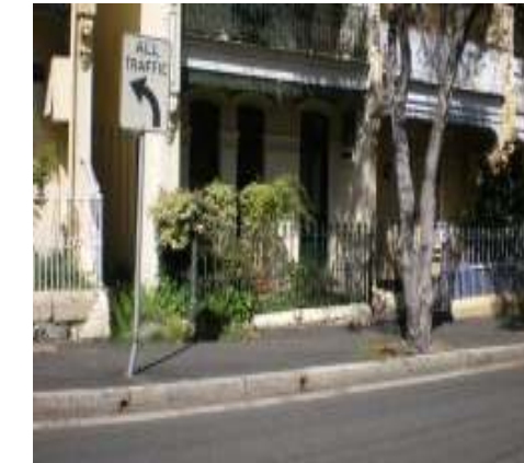
130 Underwood St Property inundated to 0.3m, and above floor flooding to 0.05m (89), property inundation to 0.2m (91).
