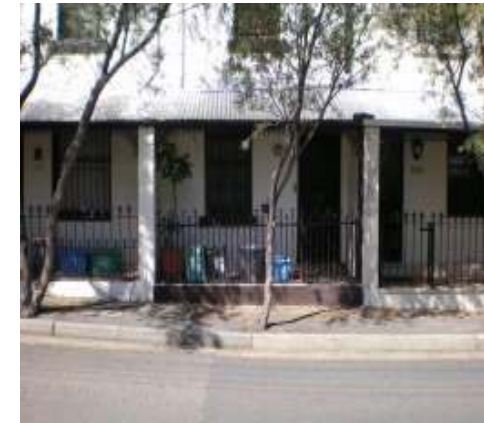
184 Underwood St Above floor flooding due to a drainage problem.
