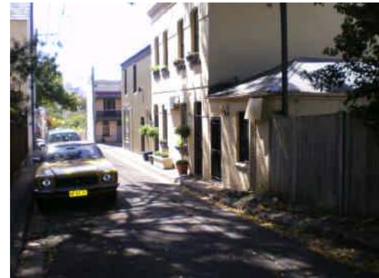
44. Ponding & Ground Floor Inundation Low point in road; possibly ponding and inundation above floor level.
