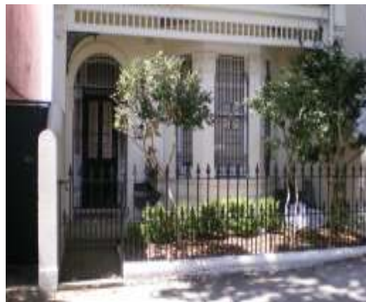
14, 28, and 30 Windsor St Inundation of below ground cellars.
