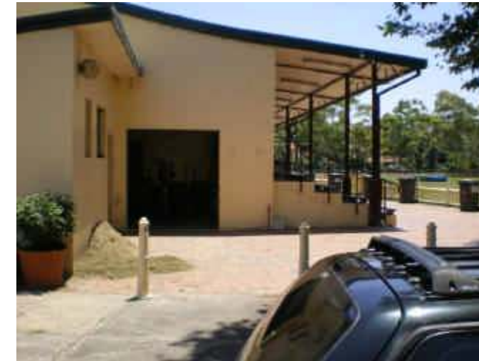
103. Ponding & Ground Floor Inundation Ponding at the end of Royston St and inundation above floor level
