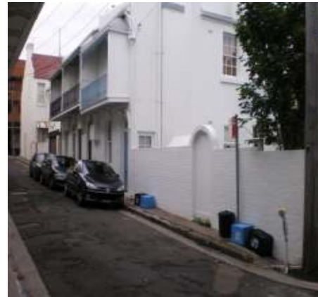
1 Tivoli St Water up to 0.08 m at front of house (89), water to 0.05 m below floor level (91).
