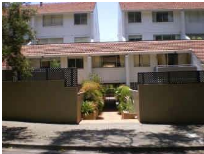
101. Other Rear of property at risk of being flooded.
