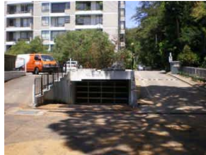
110. Garage Below Road Garage on Hampden Street at risk of being inundated.
