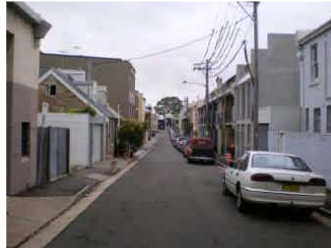
50. Ponding & Ground Floor Inundation Low point in Victoria St; possibly ponding and inundation above floor level(see 51).
