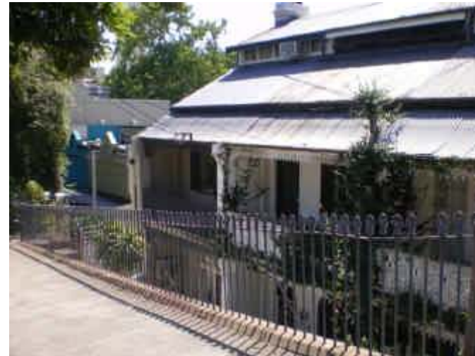
86. Floor Below Road Example of property on Cascade St at risk of being inundated.
