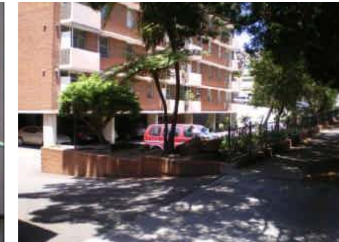
20. Garage Below Road Rear of 204 Jersey Rd
