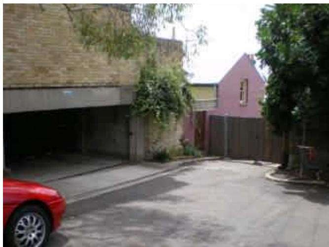
81. Ponding Gates blocking flow path down Bennetts Grove Ave
