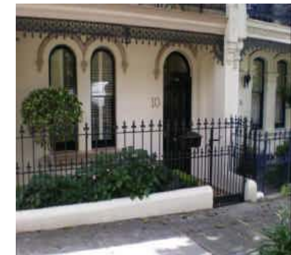
80. Ground Floor Inundation Example of property on Duxford St at risk of being inundated.
