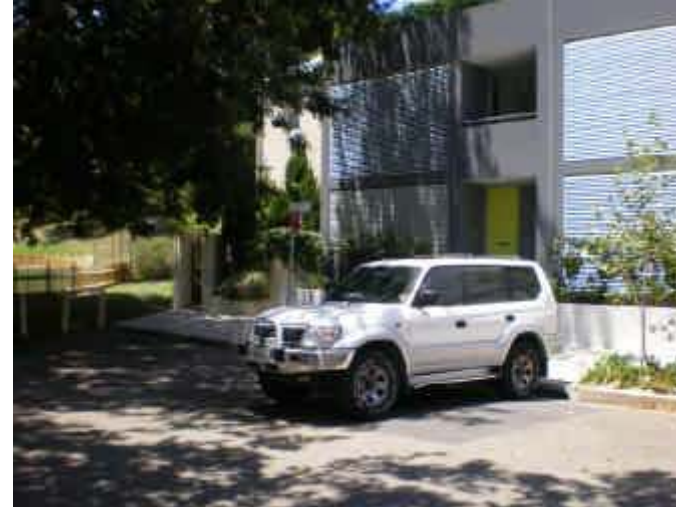
102. Ponding & Ground Floor Inundation Ponding at the end of Royston St and inundation above floor level
