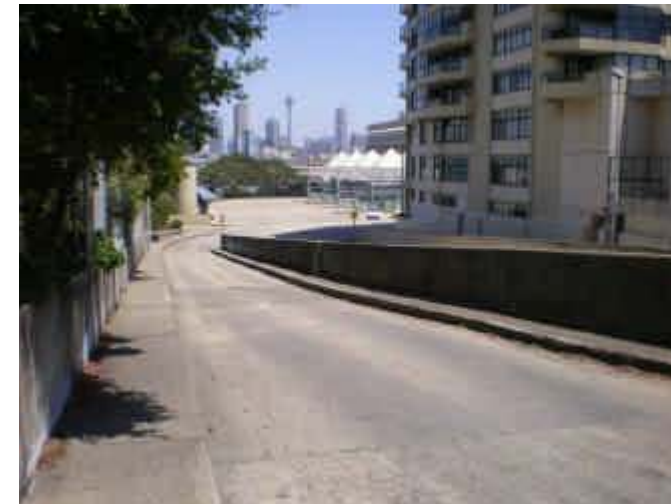
91. Other Edgecliff Station bus area at risk of being flooded by waters flowing down the ramps
