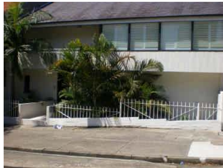
43. Floor Below Road One of several properties along Hargrave St with floor levels below road level.
