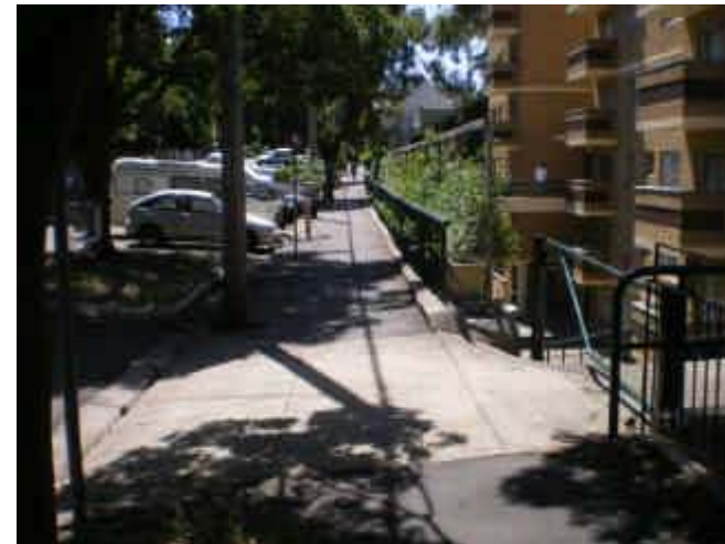
39. Ponding & Floor Below Road Low point in road
