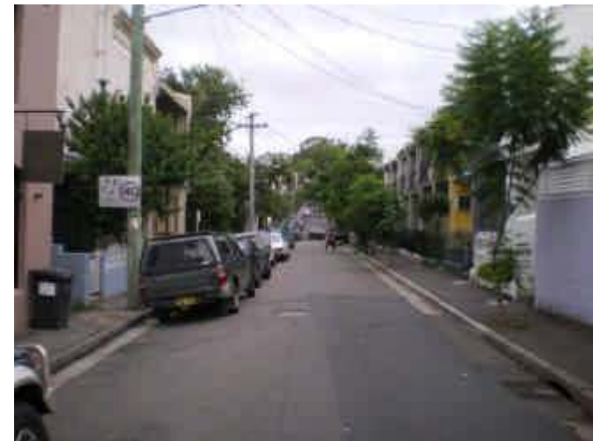
54. Ponding & Floor Below Road Low point in Underwood St(see 55).
