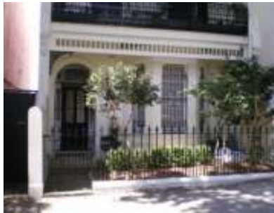
14, 28, and 30 Windsor St Inundation of below ground cellars
