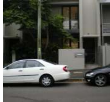
86 Holdsworth St Above floor flooding due to flows overtopping kerb in Holdsworth Street en route to Jersey Road.
