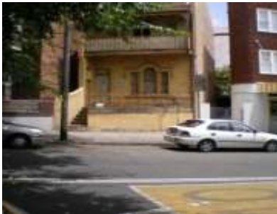
1 Gurner St Groundwater seepage due to storm events.
