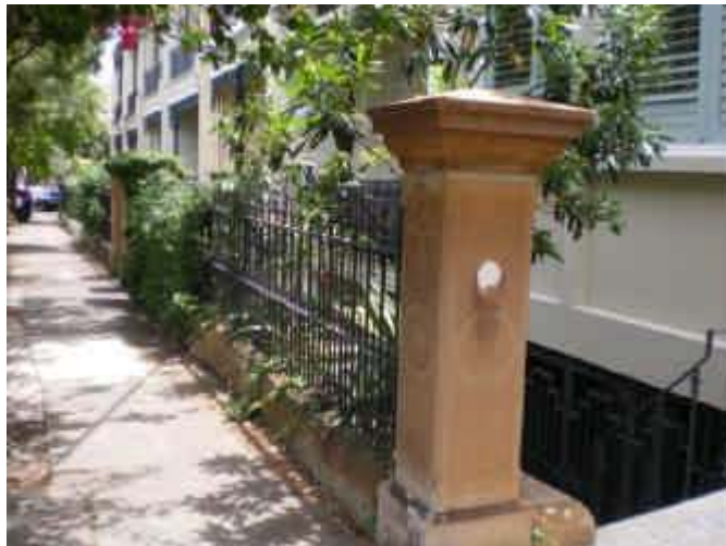
77. Floor below Road Example of property on Glenmore Rd at risk of being inundated.
