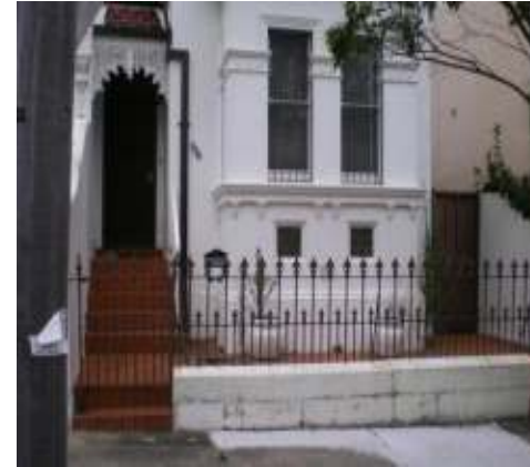
173 Windsor St Above floor level inundation.
