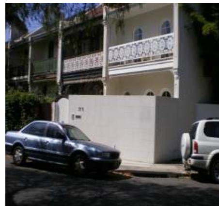
21 Paddington St Water to 0.15m below floor level.
