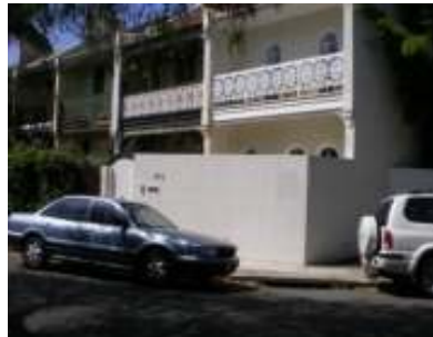
21 Paddington St Water to 0.15 below floor level.
