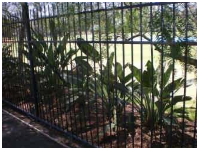
93. Flow Diversion Water could enter to the sportsground from Nield Ave
