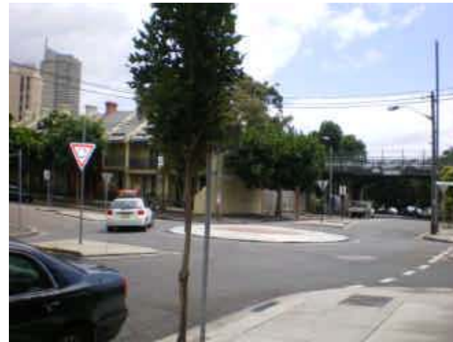
62. Ponding Intersection Campbell ave\Boundary St
