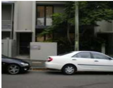
86 Holdsworth St Above floor flooding due to flows overtopping kerb in Holdsworth Street en route to Jersey Road.
