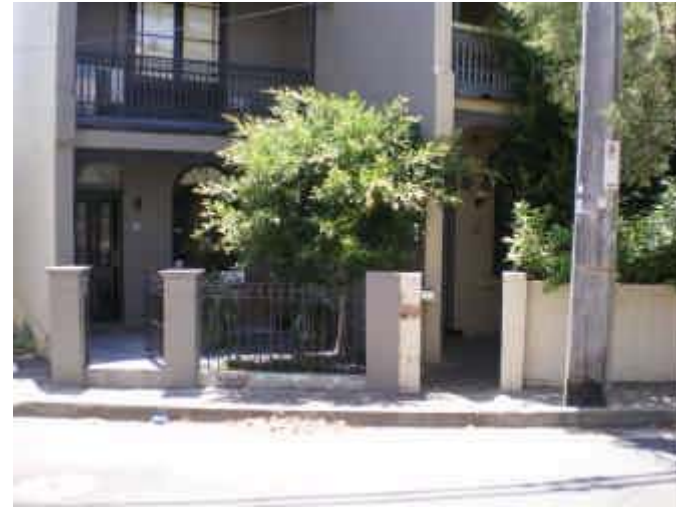
98. Ground Floor Inundation Property on Hoddle St at risk of being inundated.
