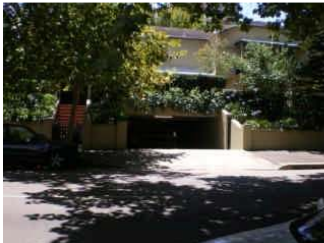
9. Garage Below Road Ocean St
