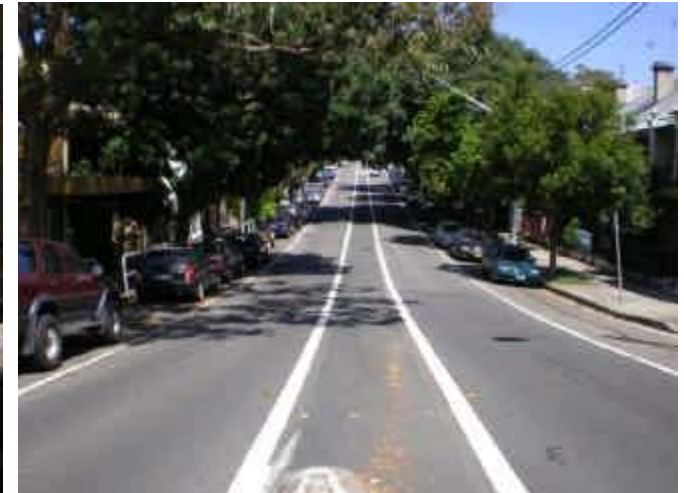
40. Ponding Low point in Hargrave St.
