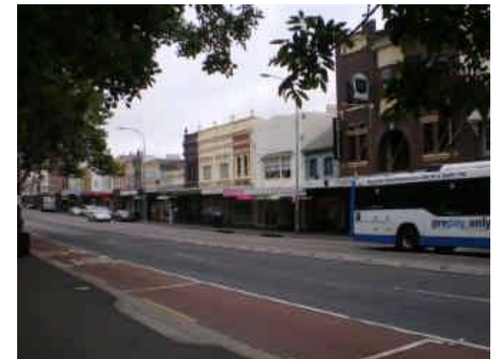
52. Ponding & Ground Floor Inundation Low point in Oxford St; possibly ponding and inundation above floor level(see 53).
