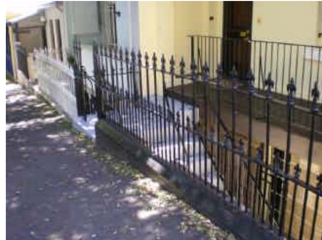
38. Floor Below Road One of several properties potentially inundated on Sutherland St
