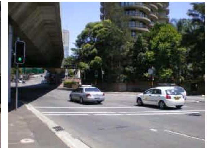
92. Ponding Intersection Nield Ave and New South Head Rd
