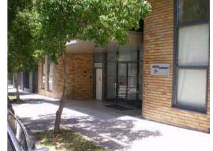
100. Floor Below Road Property on Glenmore Rd at risk of being inundated.
