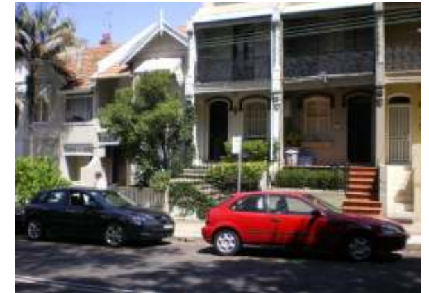
440 and 450 Glenmore Rd Above floor flooding reported, but no clear reason found.
