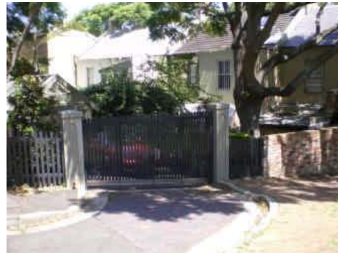
90. Ground Floor Inundation Property on Great Thorne St at risk of being inundated.
