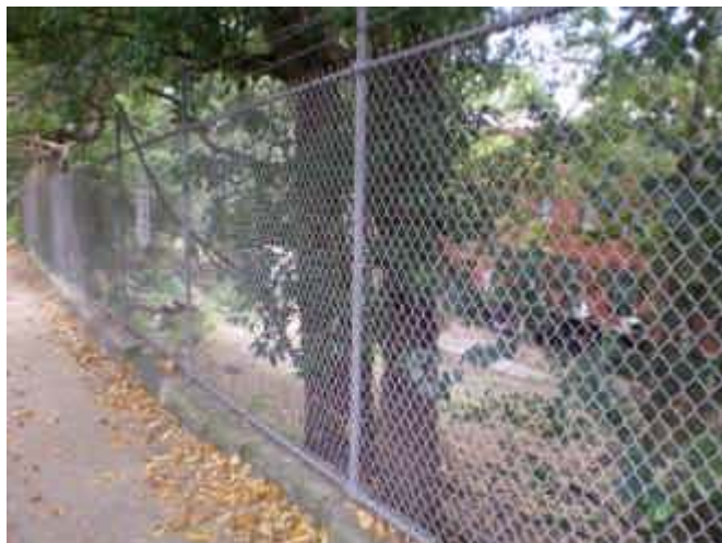
70. Garage Below Road The hospital car park could potentially be inundated by waters from Brown St.
