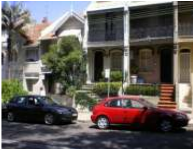
440 and 450 Glenmore Rd Above floor flooding reported, but no clear reason found.
