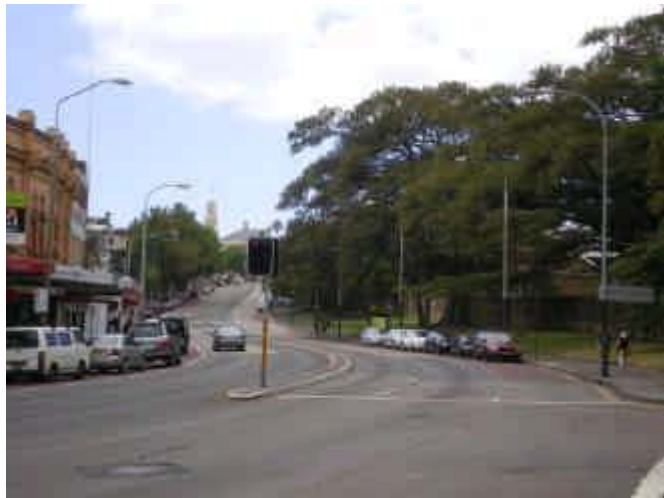
65. Ponding Low point in Oxford St. Footpath reported to have been flooded previously
