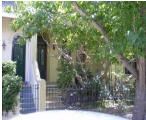
133 Windsor St Above floor flooding due to local drainage problem
