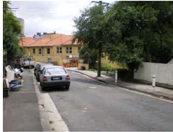
75. Ponding Low point in Cooper St. Water may flow into the reserve and down to Stephen St.
