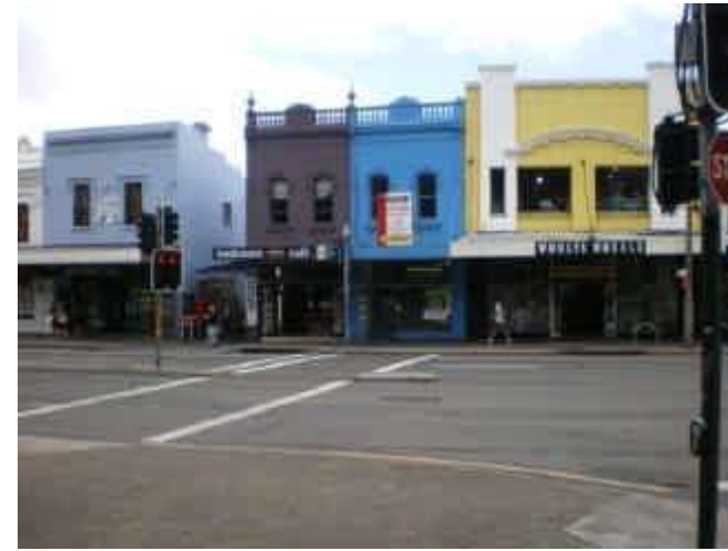
63. Ponding & Ground Floor Inundation Low point in Oxford St
