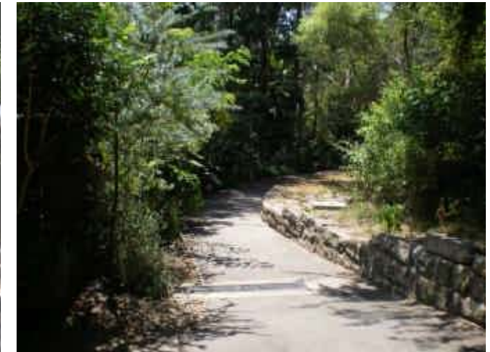
112. Flow Diversion Possible flow path from Harris St to Hampden St. (Continuation from 33)
