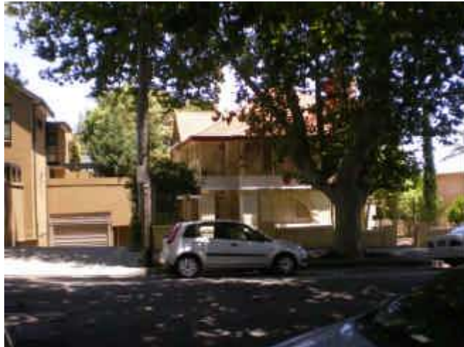
13. Garage Below Road Ocean St
