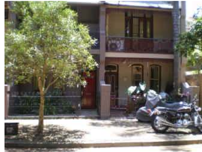
107. Ground Floor Inundation Example of properties on Cecil St at risk of inundation.
