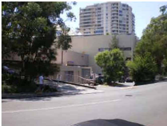
89. Garage Below Road Aldi car park/loading area at risk of being flooded
