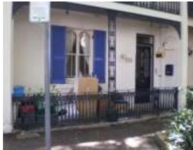
159 Paddington St Ground seepage enters residence during storms.
