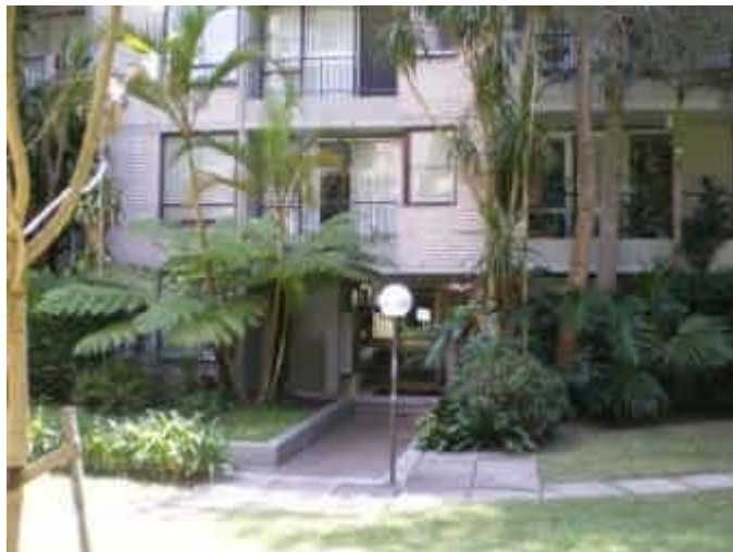
113. Ground Floor Inundation Example of property on Hampden St at risk of inundation.
