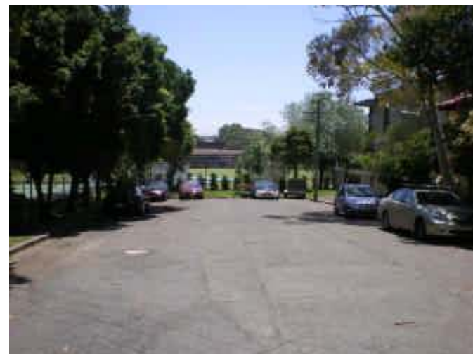
94. Ponding Possibly ponding at the end of Valoux Ave and flooding of the sportsground and adjacent properties.
