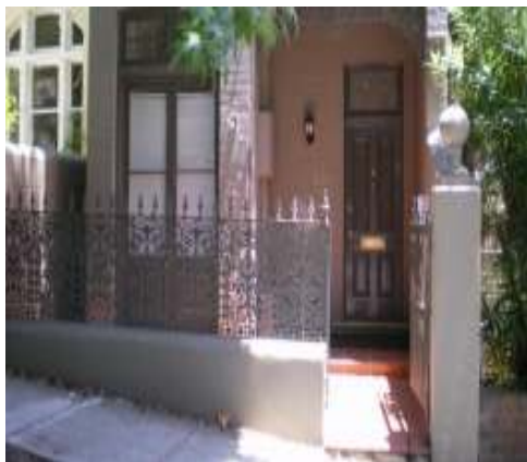
280 Glenmore Rd Groundwater seepage due to storm events.
