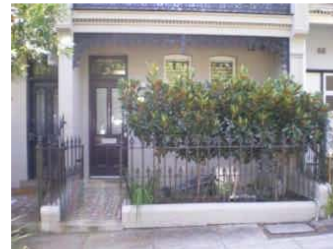
119. Ground Floor Inundation Example of property on Hopetoun St at risk of inundation.
