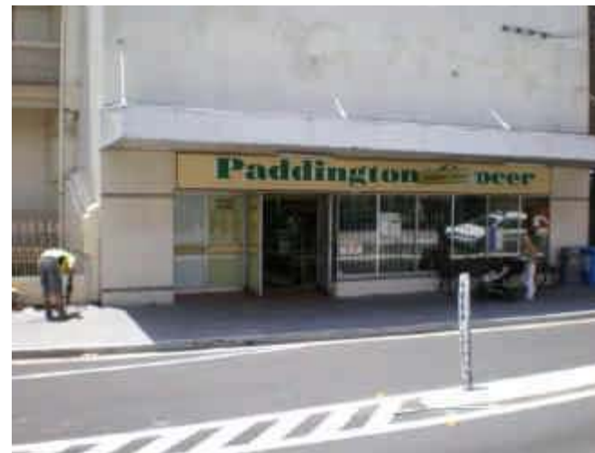
79. Ponding & Ground Floor Inundation Low point in Glenmore Rd.
