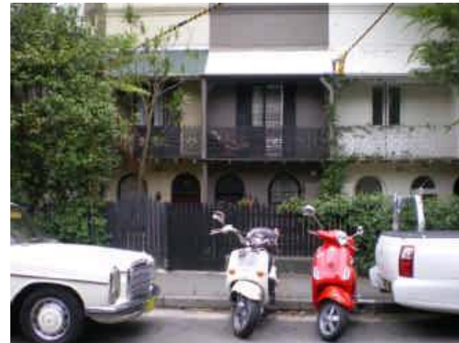
55. Floor Below Road Example of properties at risk of being inundated.
