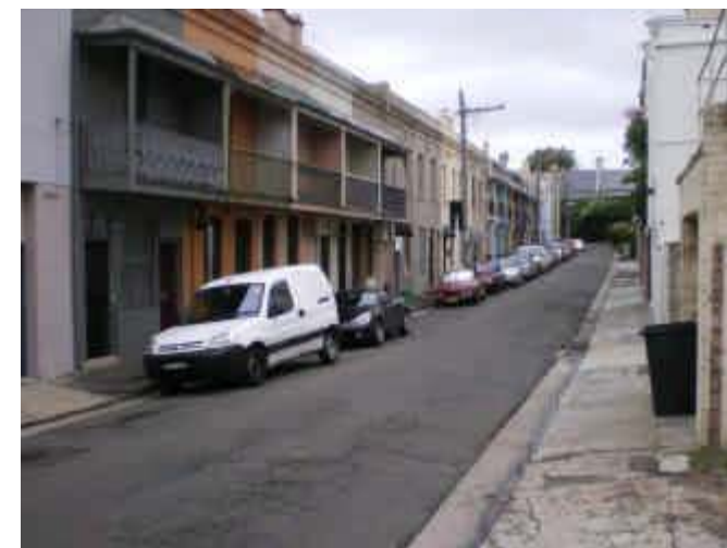
51. Ground Floor Inundation Example of house at risk of being inundated.
