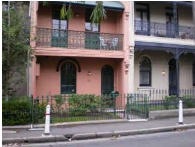
49. Ground Floor Inundation Example of house at risk of being inundated.
