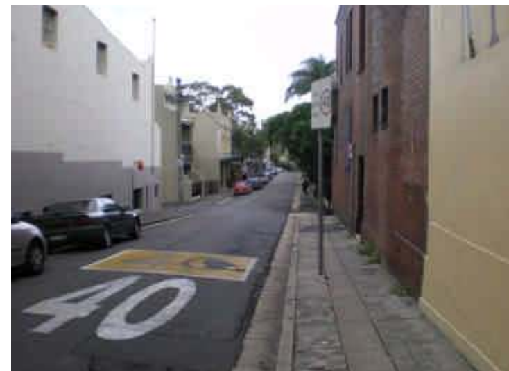
47. Ponding & Ground Floor Inundation Low point in Elizabeth St; possibly ponding and inundation above floor level(see 49).
