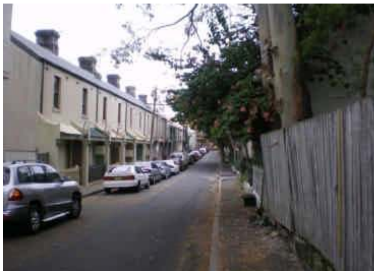
45. Ponding & Ground Floor Inundation Low point in George St; possibly ponding and inundation above floor level.
