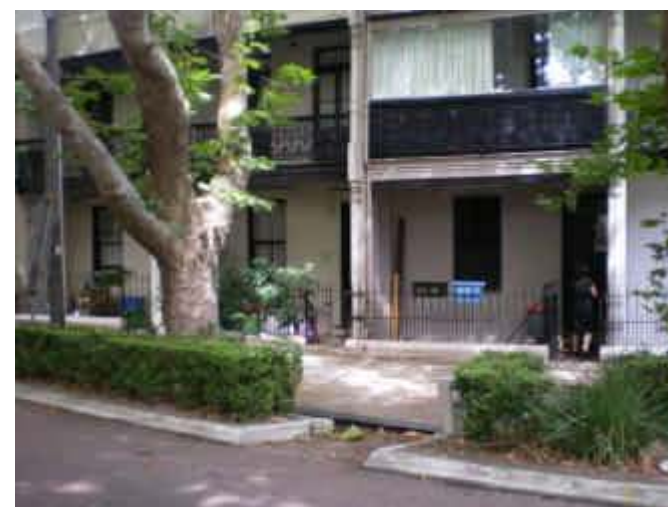
59. Floor Below Road Example of properties at risk of being inundated.
