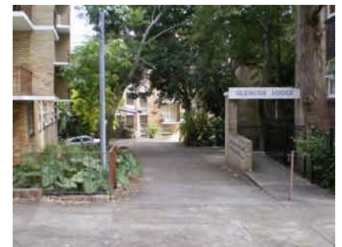
60. Garage Below Road 56 Hopewell St.
