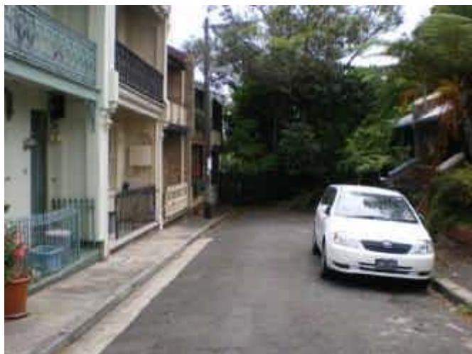
69. No Flow Path Ponding and possibly floor inundation will occur at the northern end of Prospect St.
