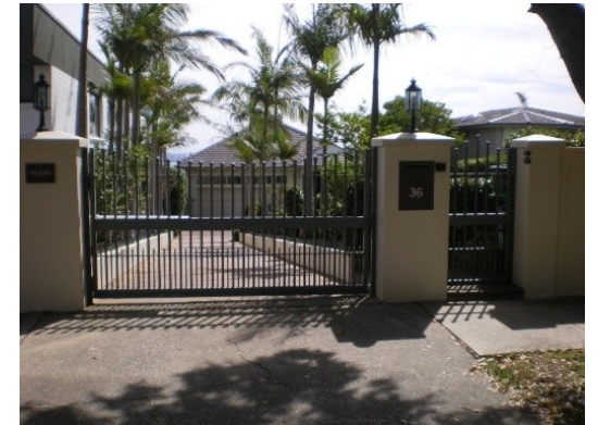
253. 36 Chamberlain Avenue Floor below road, Garage below road, Flooding due to overland flow from road above property
