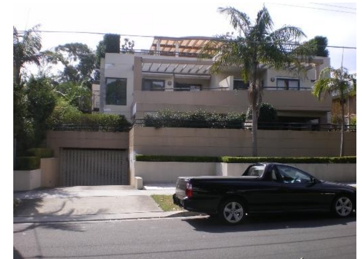
275. 18 Spencer Street Problem identified by Reference 4, field trip results show: Garage below road, High Flow along Spencer Street
