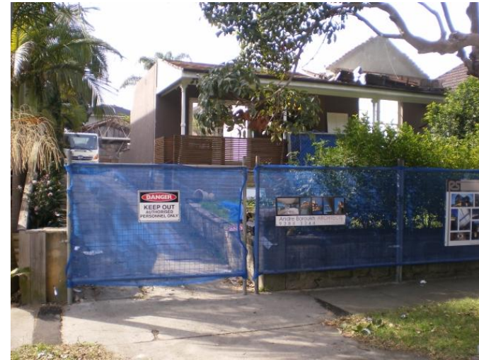
336. 58 Wilberforce Avenue Problem identified by Reference 4, field trip results show: No problem identified
