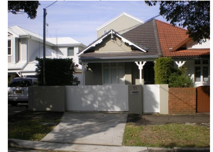
304. 11 Spencer Street Problem identified by Reference 4, field trip results show: High Flow along Spencer Street
