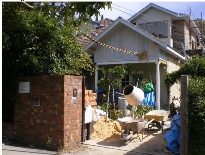
326. 61 Dover Road Problem identified by Reference 2, field trip results show: Ponding on street
