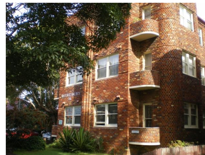
228. 23 Newcastle Street Problem identified by Reference 2, field trip results show: Very high flow and water level in nearby channel
