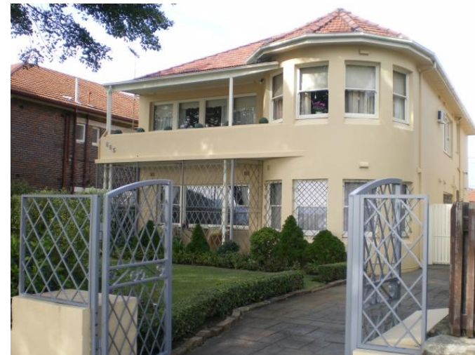
19. 665 New South Head Road Problem identified by Reference 2, field trip results show: Very high flow and water level in nearby channel
