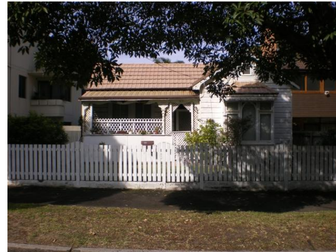
298. 23 Spencer Street Problem identified by Reference 4, field trip results show: High Flow along Spencer Street
