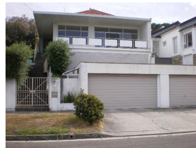
164. 60 Boronia Road Problem identified by Reference 4, field trip results show: Garage below road, Ponding on street, Flooding due to overland flow from road above property
