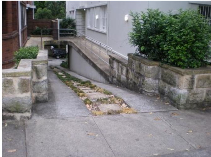
193. 78 Birriga Road Problem identified by Reference 2, field trip results show: Floor below road, Garage below road, Road and footpath graded towards residence, Main flow channel bordering residence
