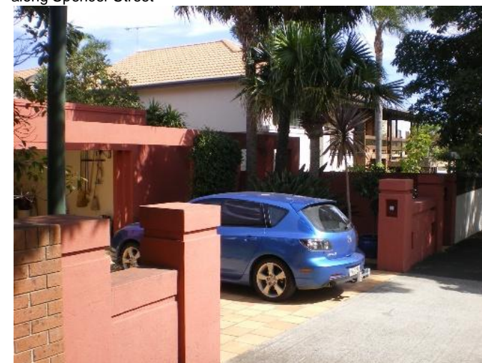
307. 3 Spencer Street Problem identified by Reference 4, field trip results show: Floor below road, Garage below road, High Flow along Spencer Street
