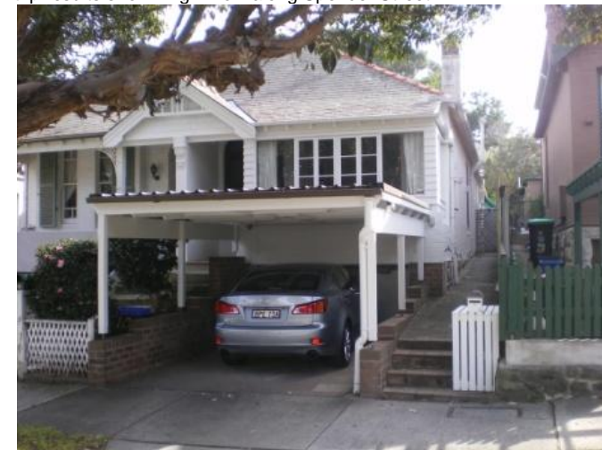
278. 12 Spencer Street Problem identified by Reference 4, field trip results show: High Flow along Spencer Street
