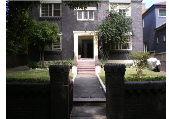
199. 267 O'Sullivan Road Problem identified by Reference 2, field trip results show: No problem identified
