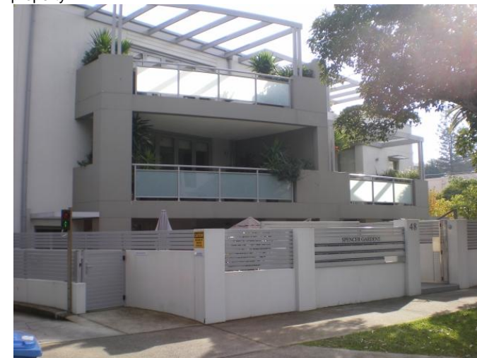
266. 48 Spencer Street Problem identified by Reference 4, field trip results show: High Flow along Spencer Street
