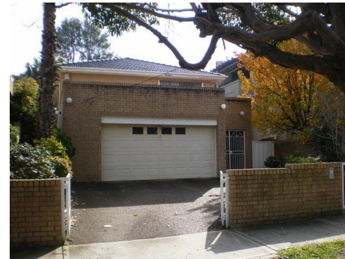
274. 22 Spencer Street Problem identified by Reference 4, field trip results show: High Flow along Spencer Street
