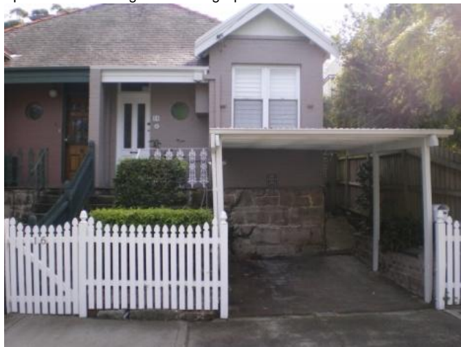
276. 16 Spencer Street Problem identified by Reference 4, field trip results show: High Flow along Spencer Street
