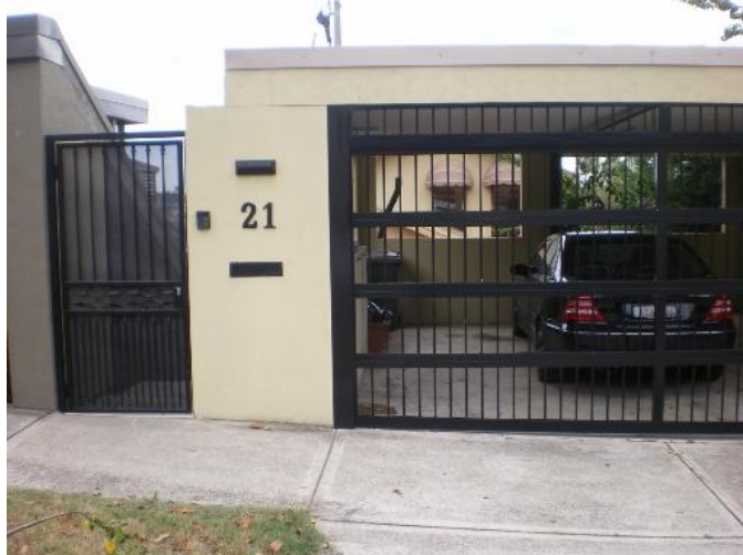
173. 21 Bundarra Road Problem identified by Reference 4, field trip results show: Floor below road, Garage below road, Flooding due to overland flow from road above property
