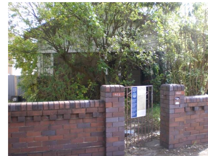
219. 482 Old South Head Road Problem identified by Reference 4, field trip results show: Very high flow and water level in nearby channel
