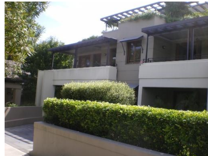
273. 24 Spencer Street Problem identified by Reference 4, field trip results show: High Flow along Spencer Street
