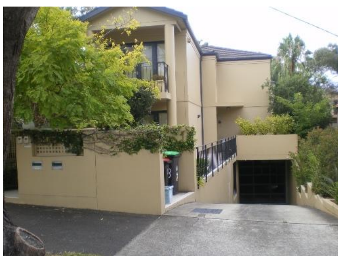
293. 35 Spencer Street Problem identified by Reference 4, field trip results show: Garage below road, Flow diversion, High Flow along Spencer Street
