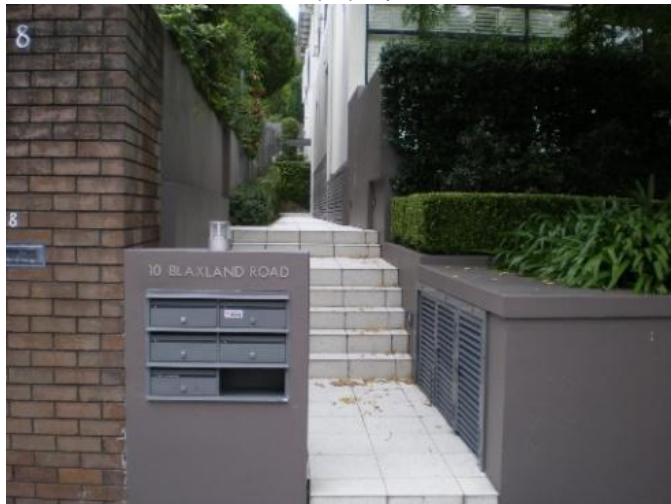
182. 10 Blaxland Road Problem identified by Reference 4, field trip results show: Floor below road, Garage below road, High velocity flow, Flooding due to overland flow path from adjacent street
