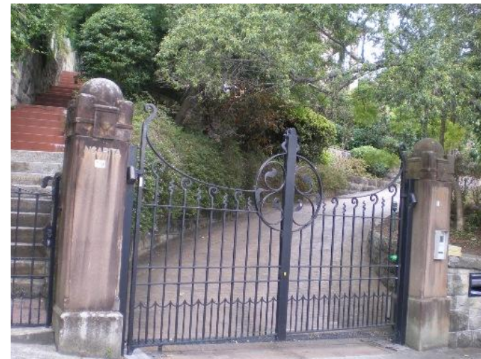
7. 17 Cranbrook Road Problem identified by Reference 4, field trip results show: Flooding due to overland flow from road above property,
