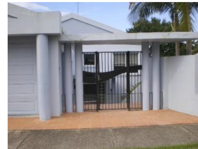
158. 49 Boronia Road Problem identified by Reference 2, field trip results show: Floor below road, Ponding on street, Flooding due to overland flow from road above property
