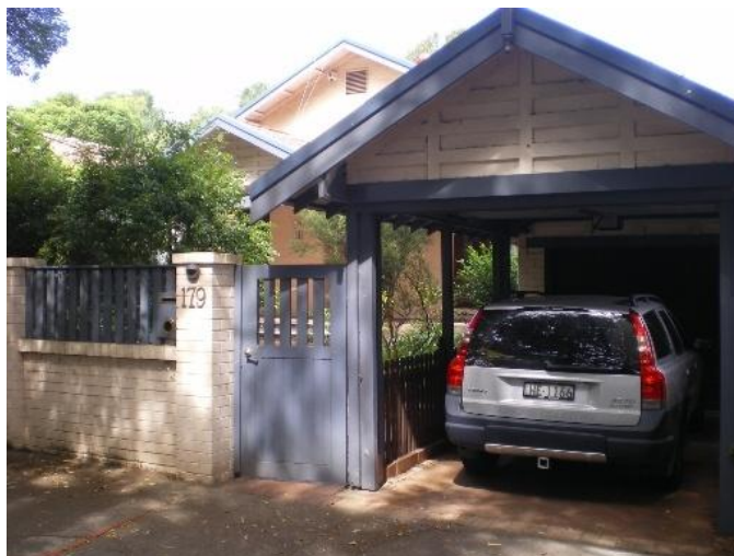
149. 179 O'Sullivan Road Problem identified by Reference 4, field trip results show: Flooding due to overland flow from road above property
