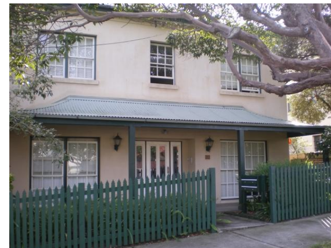
270. 32 Spencer Street Problem identified by Reference 4, field trip results show: High Flow along Spencer Street
