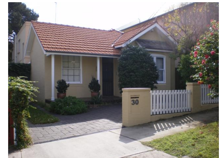
271. 30 Spencer Street Problem identified by Reference 4, field trip results show: High Flow along Spencer Street
