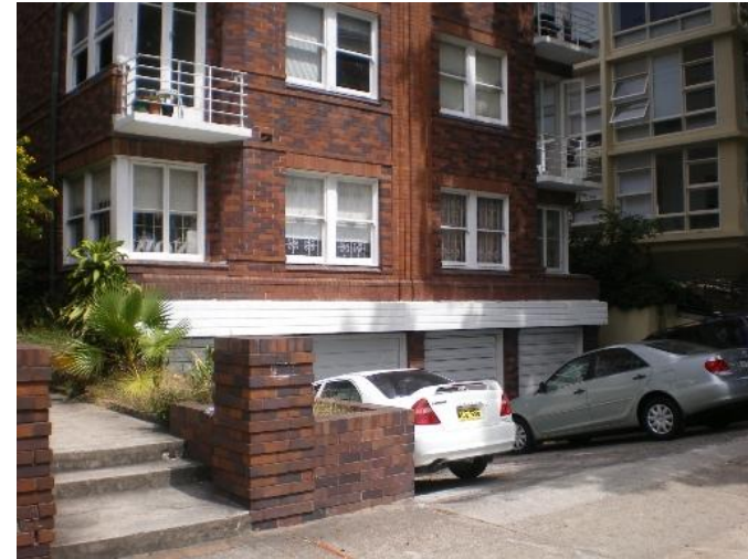
1. 595 New South Head Road Problem identified by Reference 2, field trip results show: Garage below road
