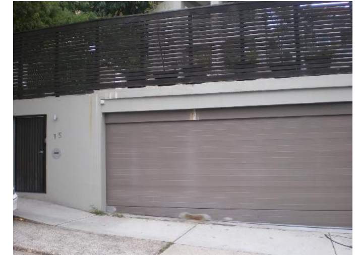
5. 15 Cranbrook Road Problem identified by Reference 4, field trip results show: Flooding due to overland flow from road above property,
