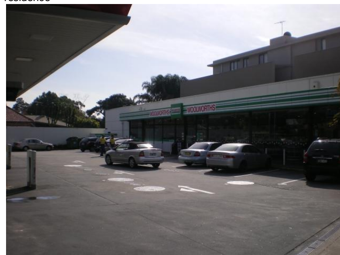
221. 488 Old South Head Road Problem identified by Reference 4, field trip results show: Very high flow and water level in nearby channel
