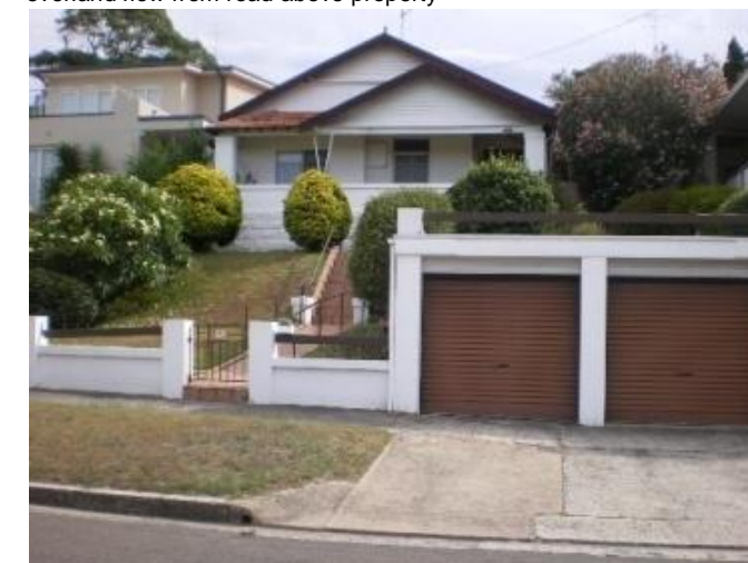
165. 58 Boronia Road Problem identified by Reference 4, field trip results show: Garage below road, Ponding on street, Flooding due to overland flow from road above property
