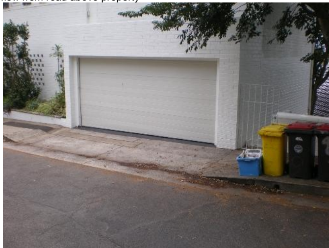
6. 9 Cranbrook Lane Problem identified by Reference 4, field trip results show: Floor below road, Garage below road, Main flow channel bordering residence, Ponding on street, Flooding due to overland flow from road above property
