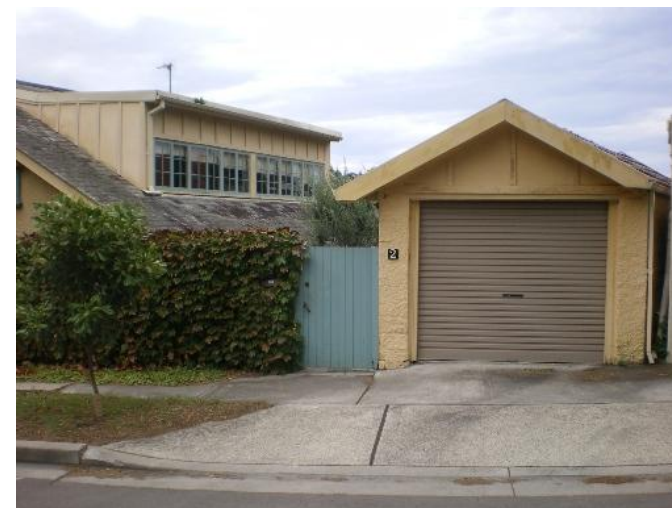
47. 2 Beresford Crescent Problem identified by Reference 4, field trip results show: Floor below road, Garage below road, Ponding on street
