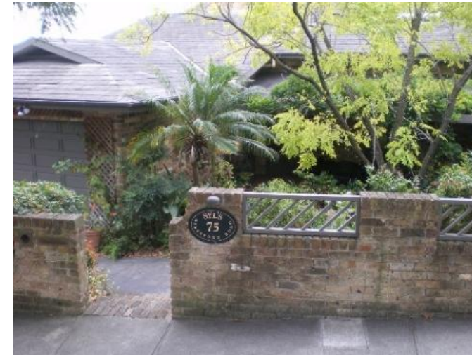
91. 75 Beresford Road Problem identified by Reference 2, field trip results show: Floor below road, Garage below road, Main flow channel bordering residence
