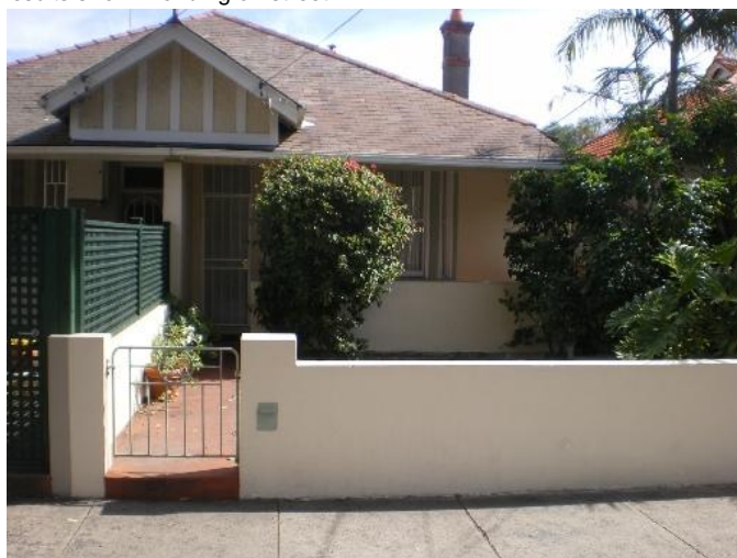
330. 53 Dover Road Problem identified by Reference 4, field trip results show: Ponding on street
