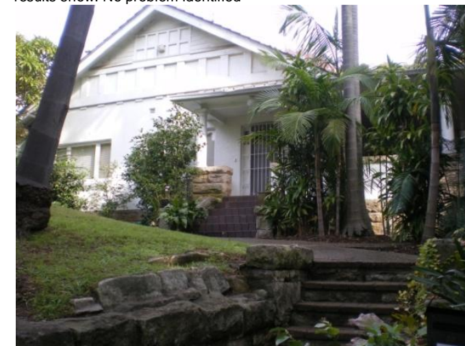
44. 50 Beresford Road Problem identified by Reference 4, field trip results show: Flooding due to overland flow from road above property
