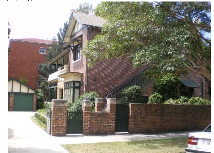
15. 3 Balfour Road Problem identified by Reference 2, field trip results show: No problem identified
