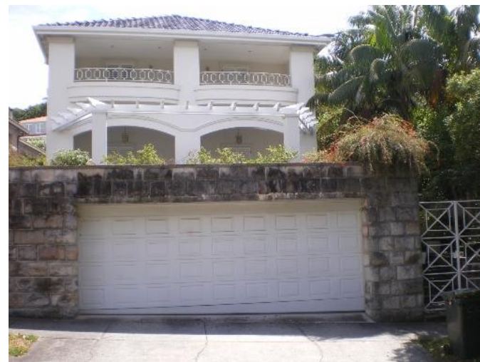
46. 56 Beresford Road Problem identified by Reference 4, field trip results show: Flooding due to overland flow from road above property
