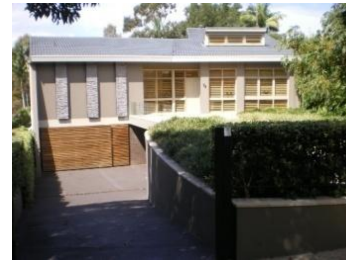
81. 74 Salisbury Road Problem identified by Reference 3, field trip results show: Floor below road, Garage below road, Main flow channel bordering residence
