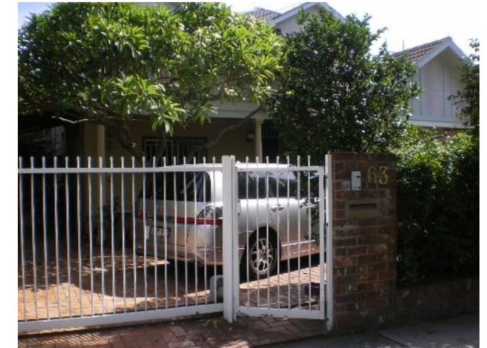
325. 63 Dover Road Problem identified by Reference 2, field trip results show: Ponding on street
