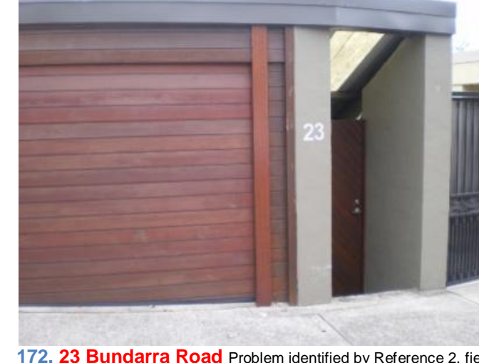
172. 23 Bundarra Road Problem identified by Reference 2, field trip results show: Floor below road, Garage below road
