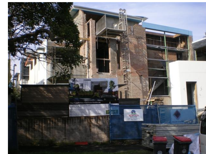
288. 47 Spencer Street Problem identified by Reference 4, field trip results show: High Flow along Spencer Street
