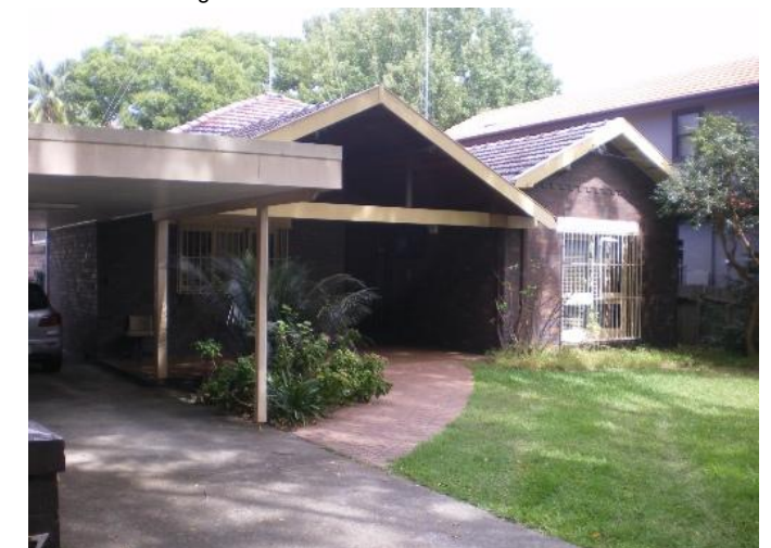
148. 177 O'Sullivan Road Problem identified by Reference 4, field trip results show: Floor below road, Flooding due to overland flow from road above property
