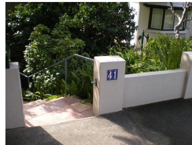
155. 41 Boronia Road Problem identified by Reference 2, field trip results show: Ponding on street
