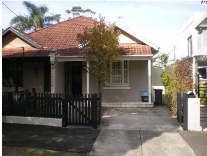
301. 17 Spencer Street Problem identified by Reference 4, field trip results show: High Flow along Spencer Street
