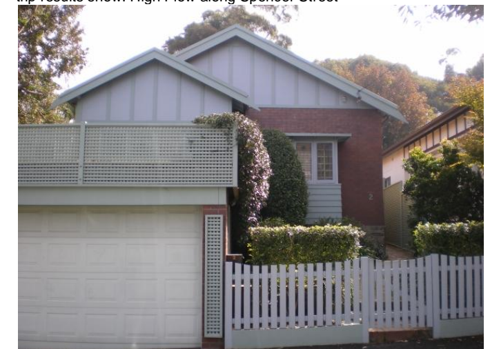
283. 2 Spencer Street Problem identified by Reference 4, field trip results show: High Flow along Spencer Street
