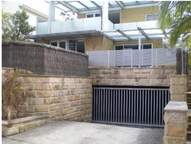
335. 56 Wilberforce Avenue Problem identified by Reference 4, field trip results show: Garage below road, Flooding due to overland flow from road above property
