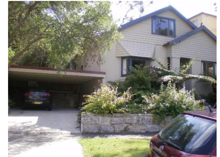
261. 14 Mitchell Road Problem identified by Reference 2, field trip results show: Flooding due to overland flow from road above property
