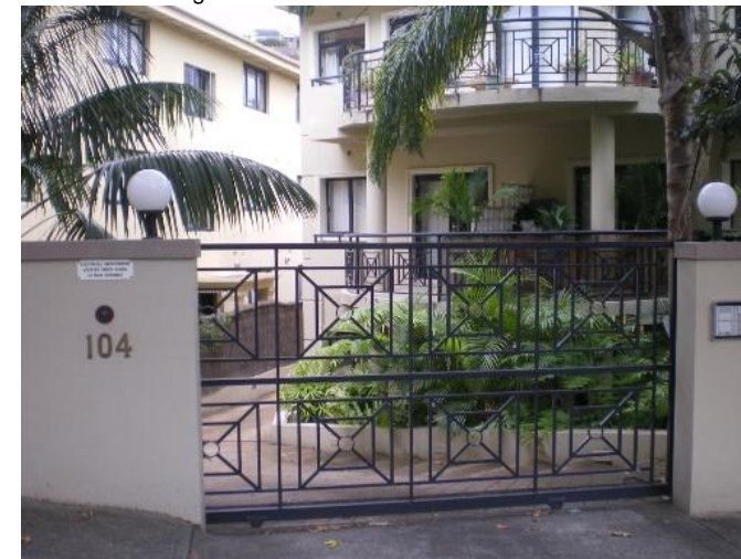
102. 104 Balfour Road Problem identified by Reference 3, field trip results show: Floor below road, Yard flooding likely
