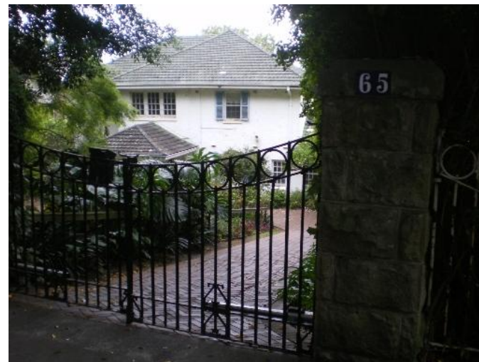
55. 65 Victoria Road Problem identified by Reference 4, field trip results show: Floor below road, Ponding on street, No flow path
