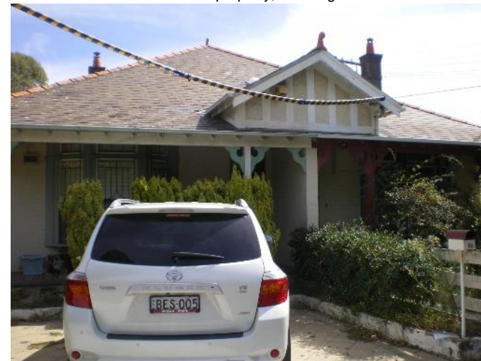
327. 59 Dover Road Problem identified by Reference 2, field trip results show: Ponding on street
