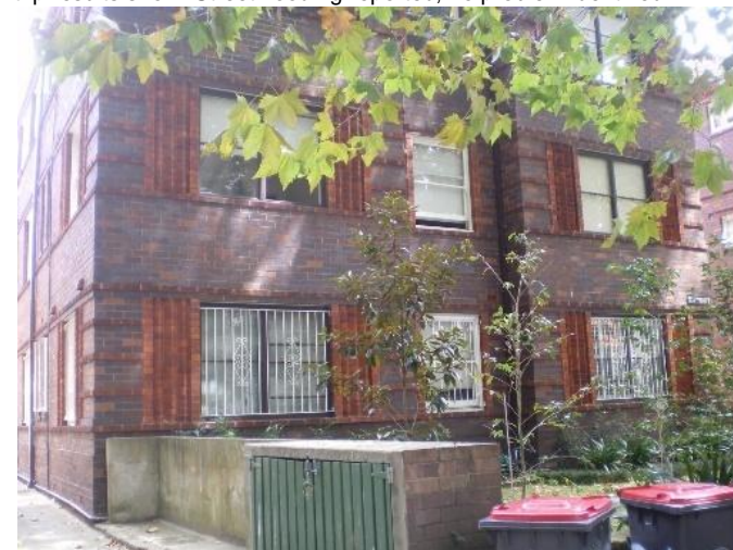
35. 26 Balfour Road Problem identified by Reference 4, field trip results show: No problem identified
