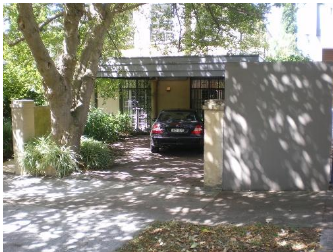
76. 60 Salisbury Road Problem identified by Reference 3, field trip results show: Floor below road, Garage below road, Main flow channel bordering residence
