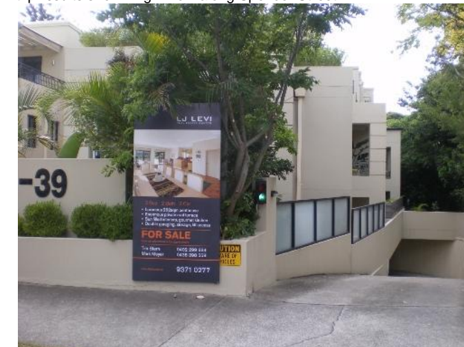
292. 37 Spencer Street Problem identified by Reference 4, field trip results show: Floor below road, Garage below road, High Flow along Spencer Street
