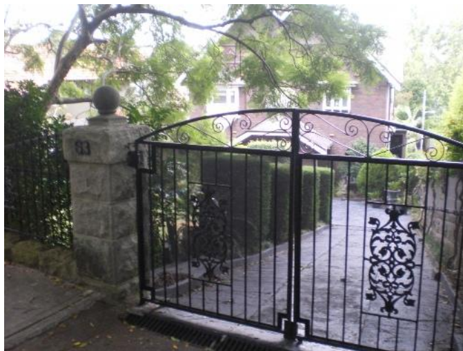
54. 63 Victoria Road Problem identified by Reference 4, field trip results show: Floor below road, Ponding on street, No flow path
