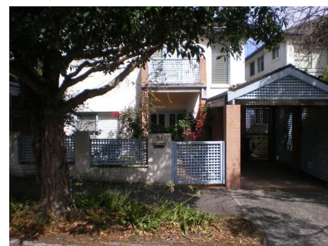
295. 31 Spencer Street Problem identified by Reference 4, field trip results show: Floor below road, Garage below road, High Flow along Spencer Street
