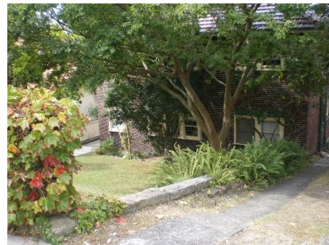
129. 55 Latimer Road Problem identified by Reference 3, field trip results show: Flooding due to overland flow from road above property
