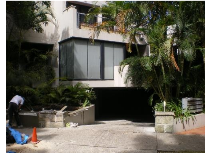
198. 271 O'Sullivan Road Problem identified by Reference 2, field trip results show: Garage below road
