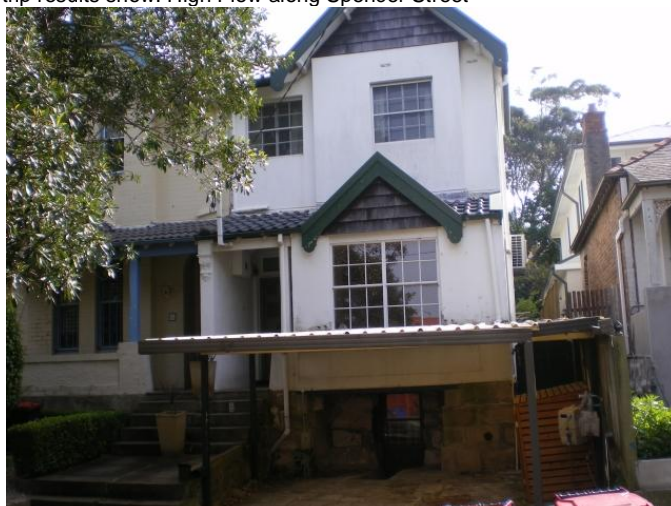
280. 8 Spencer Street Problem identified by Reference 4, field trip results show: High Flow along Spencer Street
