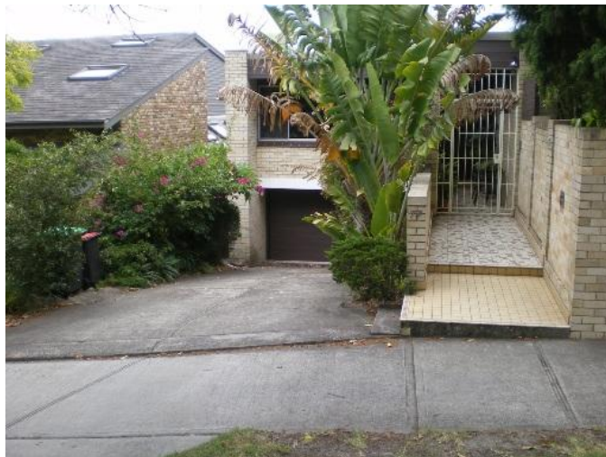
93. 77 Beresford Road Problem identified by Reference 2, field trip results show: Garage below road, Main flow channel bordering residence
