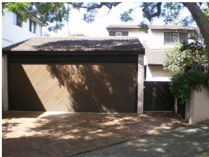
122. 75 Balfour Road Problem identified by Reference 3, field trip results show: Floor below road, Garage below road, Main flow channel bordering residence
