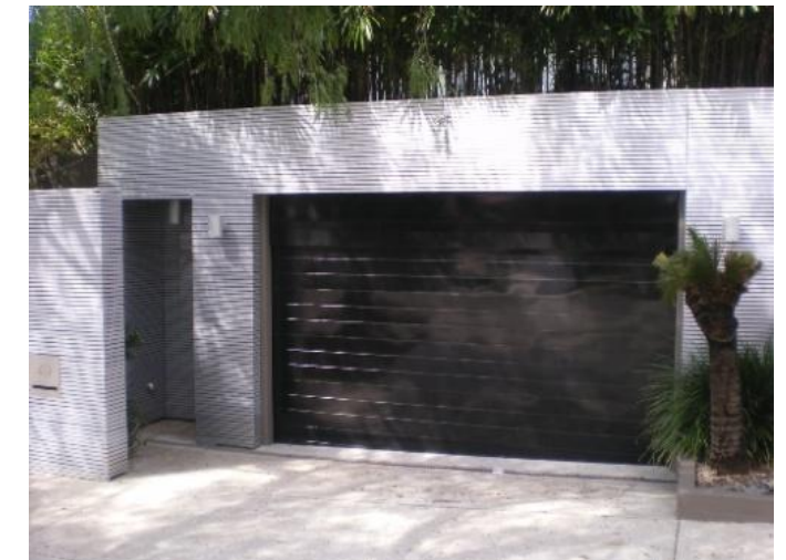
118. 49 Balfour Road Problem identified by Reference 3, field trip results show: Floor below road, Garage below road, Main flow channel bordering residence
