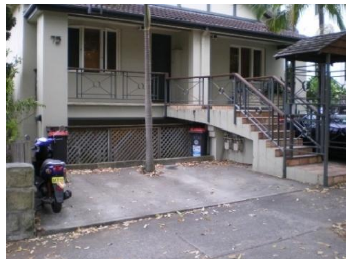
205. 75 Birriga Road Problem identified by Reference 2, field trip results show: Floor below road, Road and footpath graded towards residence
