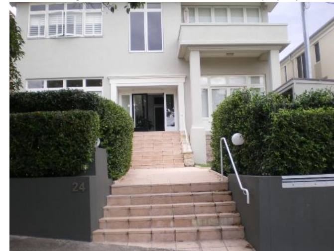
184. 22 Blaxland Road Problem identified by Reference 2, field trip results show: Flooding due to overland flow from road above property
