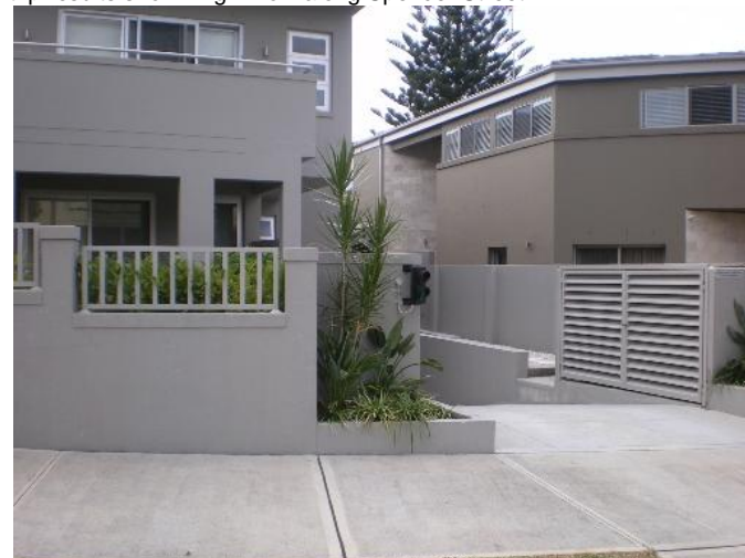
290. 43 Spencer Street Problem identified by Reference 4, field trip results show: Garage below road, High Flow along Spencer Street
