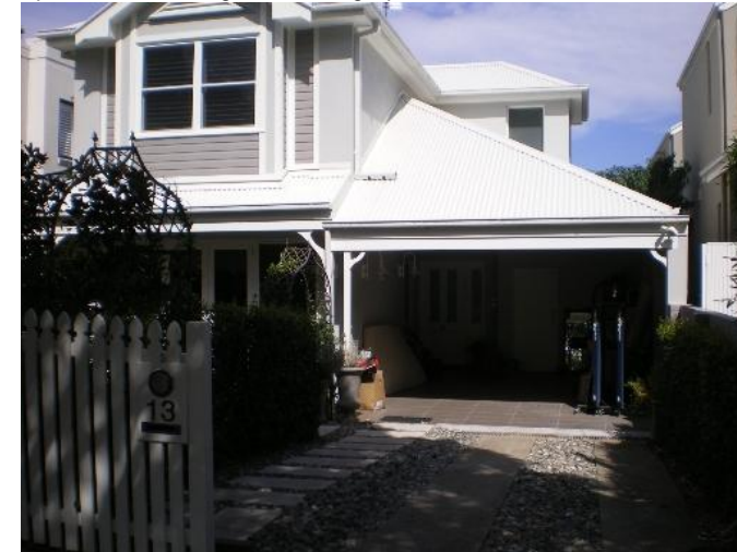
303. 13 Spencer Street Problem identified by Reference 4, field trip results show: Floor below road, Garage below road, High Flow along Spencer Street
