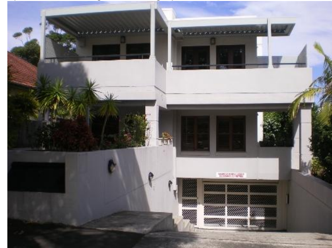
302. 15 Spencer Street Problem identified by Reference 4, field trip results show: Garage below road, High Flow along Spencer Street
