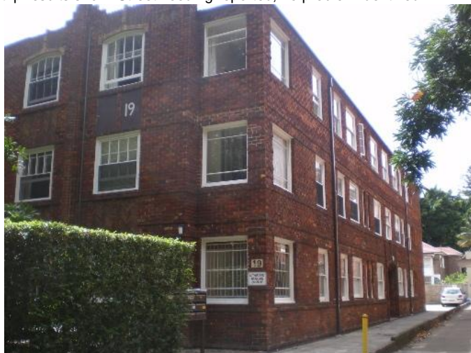
33. 19 Balfour Road Problem identified by Reference 4, field trip results show: No problem identified
