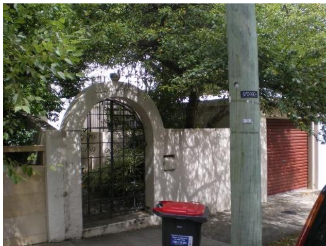
202. 245 O'Sullivan Road Problem identified by Reference 2, field trip results show: Flooding due to overland flow from road above property
