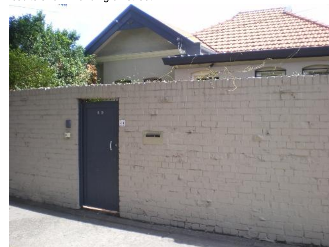
332. 49 Dover Road Problem identified by Reference 2, field trip results show: Ponding on street
