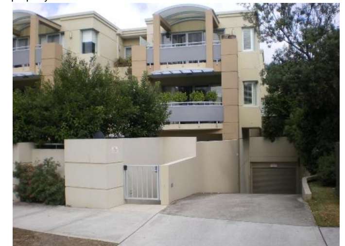
267. 44 Spencer Street Problem identified by Reference 4, field trip results show: High Flow along Spencer Street
