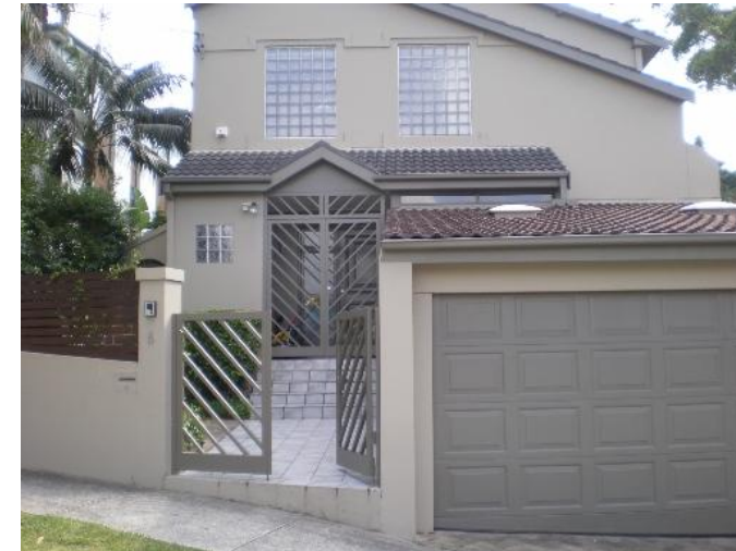
259. 6 Mitchell Road Problem identified by Reference 2, field trip results show: Flooding due to overland flow from road above property
