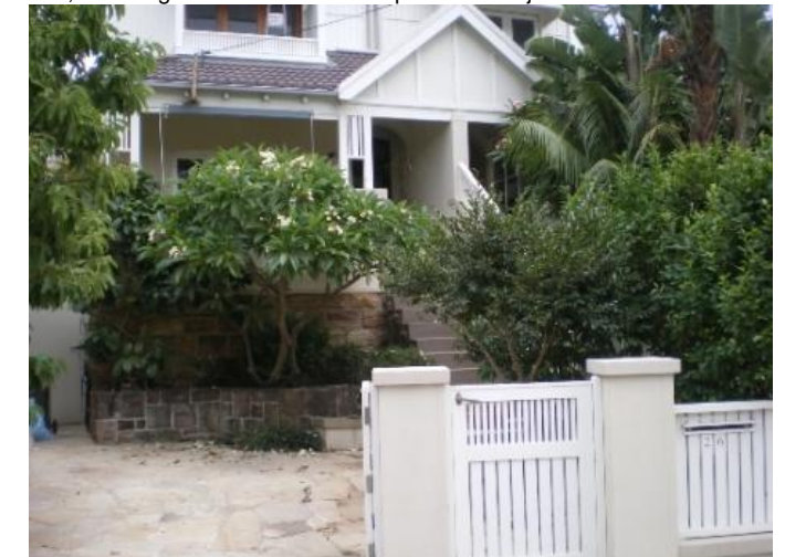
185. 26 Blaxland Road Problem identified by Reference 2, field trip results show: Flooding due to overland flow from road above property
