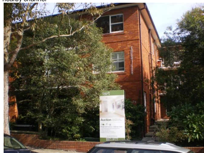
227. 39 Newcastle Street Problem identified by Reference 2, field trip results show: Garage below road
