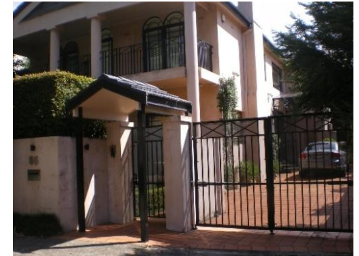
92. 86 Balfour Road Problem identified by Reference 2, field trip results show: Flooding due to overland flow from road above property
