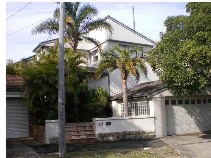
287. 49 Spencer Street Problem identified by Reference 4, field trip results show: High Flow along Spencer Street
