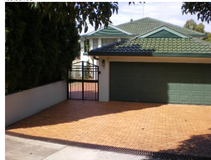
80. 72 Salisbury Road Problem identified by Reference 2, field trip results show: Floor below road, Garage below road, Main flow channel bordering residence
