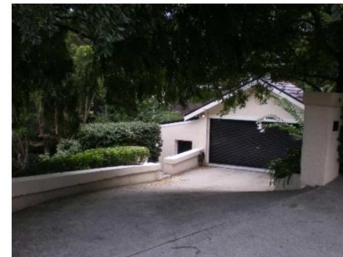
53. 52 Cranbrook Road Problem identified by Reference 2, field trip results show: Floor below road, Garage below road, Road and footpath graded towards residence
