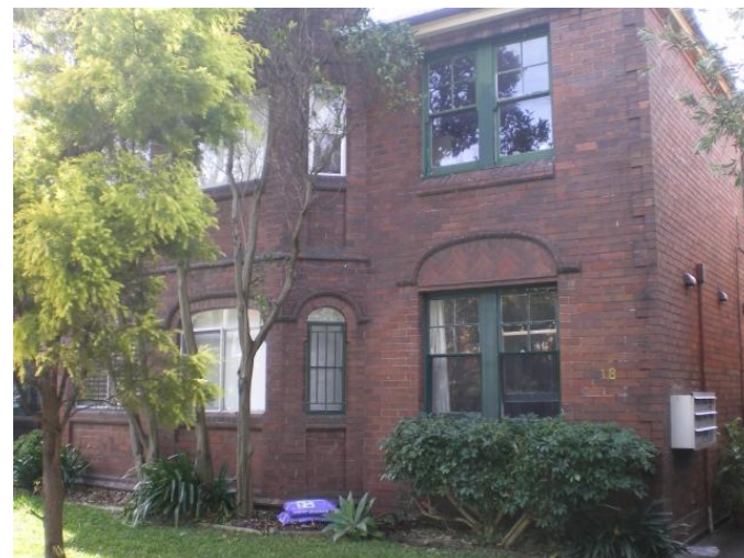
23. 18 Manion Avenue Problem identified by Reference 3, field trip results show: Street flooding reported, no problem identified
