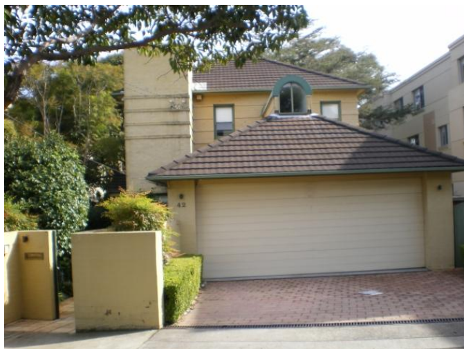
268. 42 Spencer Street Problem identified by Reference 4, field trip results show: High Flow along Spencer Street
