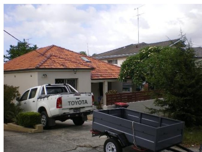
294. 33 Spencer Street Problem identified by Reference 4, field trip results show: Floor below road, Flow diversion, High Flow along Spencer Street
