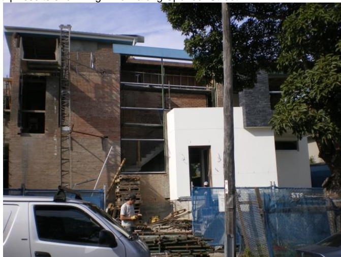
289. 45 Spencer Street Problem identified by Reference 4, field trip results show: High Flow along Spencer Street
