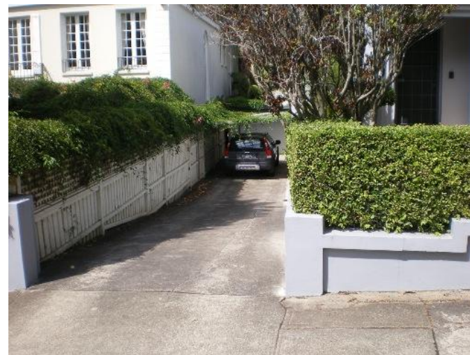
78. 68 Salisbury Road Problem identified by Reference 2, field trip results show: Floor below road, Garage below road, Main flow channel bordering residence,
