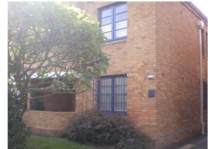
21. 8 Manion Avenue Problem identified by Reference 3, field trip results show: Street flooding reported, no problem identified
