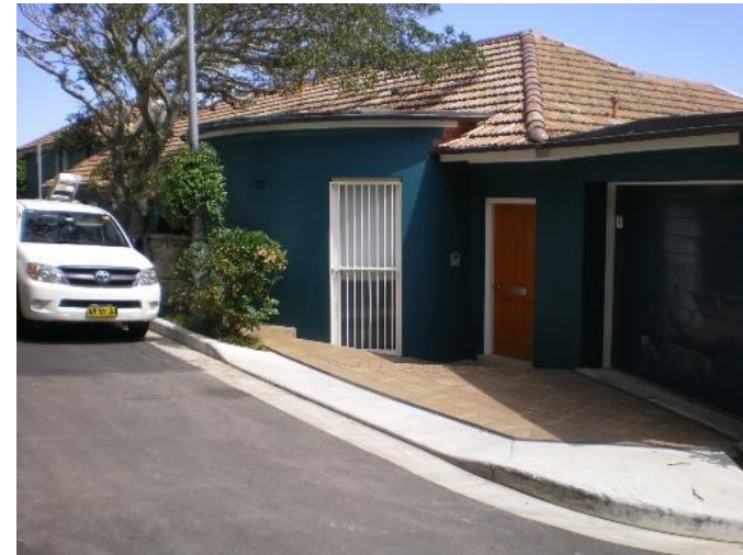
248. 8 Bayview Hill Road Problem identified by Reference 2, field trip results show: Floor below road, Road and footpath graded towards residence, Main flow channel bordering residence
