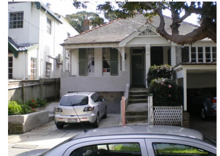
279. 10 Spencer Street Problem identified by Reference 4, field trip results show: High Flow along Spencer Street
