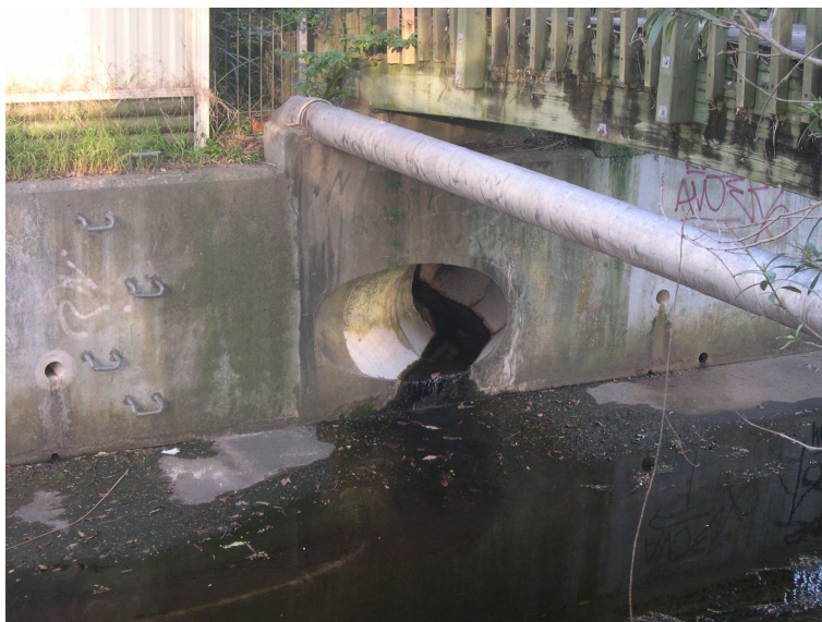
FIGURE 6.5 – Pipe Outlet Joining SWC32
