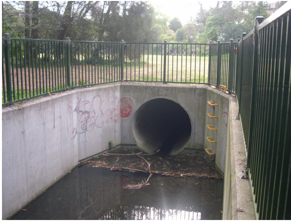
a. Culvert entrance at Cooper Park (looking downstream)
