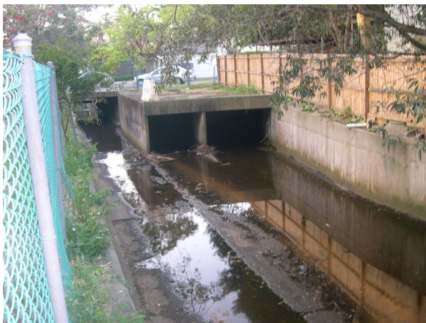
b. "2 nd amplification" culvert entrance near Carlotta Road (looking downstream)
