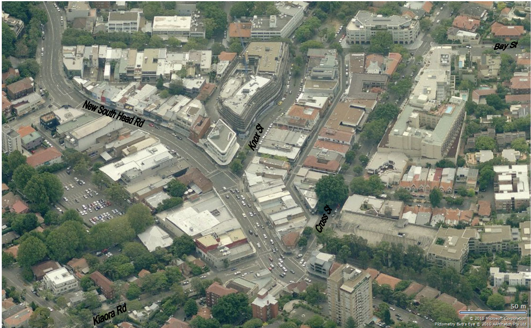
FIGURE 2.2 – Double Bay Commercial Area, looking west
