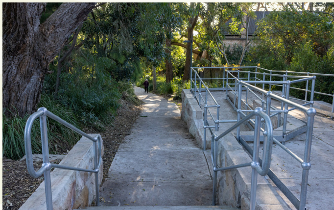
Trumper Park path upgrades for disabled access
