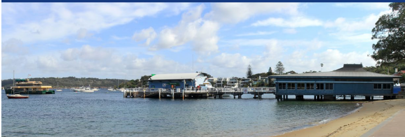
The existing Watsons Bay Wharf
