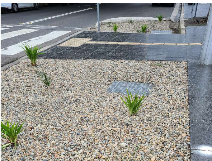
Raingarden installation at pedestrian crossing
