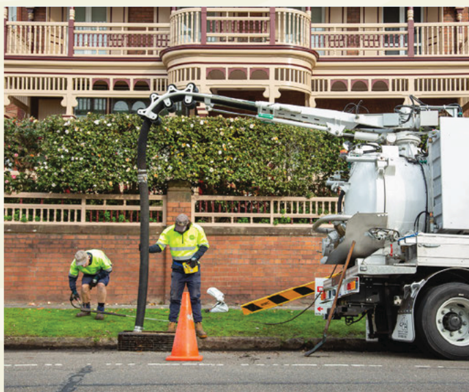
Stormwater works utilising the hydro-pump truck
