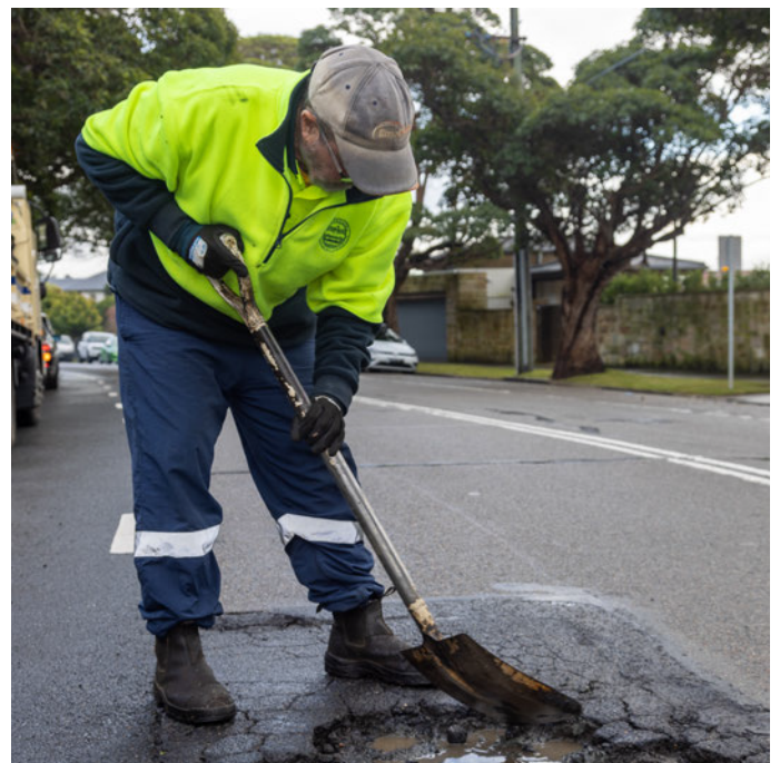
Civil Operations staff undertaking pothole repairs
