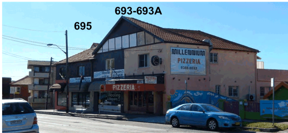
Figure 15: Existing development at 693-693A and 695 Old South Head Road, opposite the site in Waverley LGA, showing a 2 storey mixed use (retail and residential) buildings
