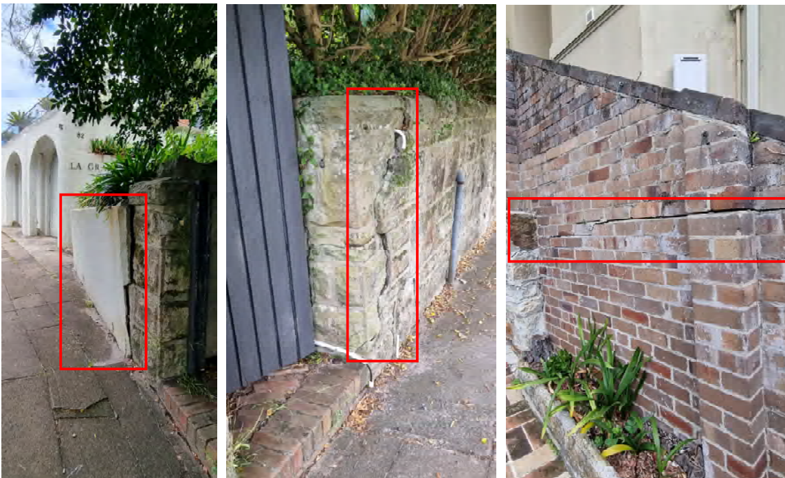
Figure 22 Brick/block retaining walls
