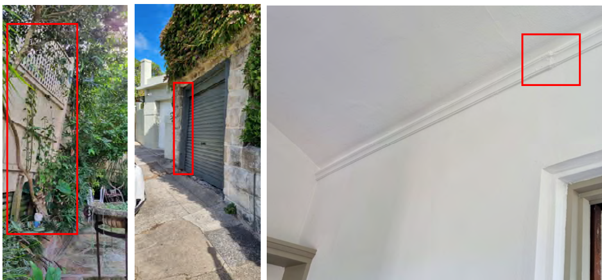
Figure 25 Timber fence and garage door
