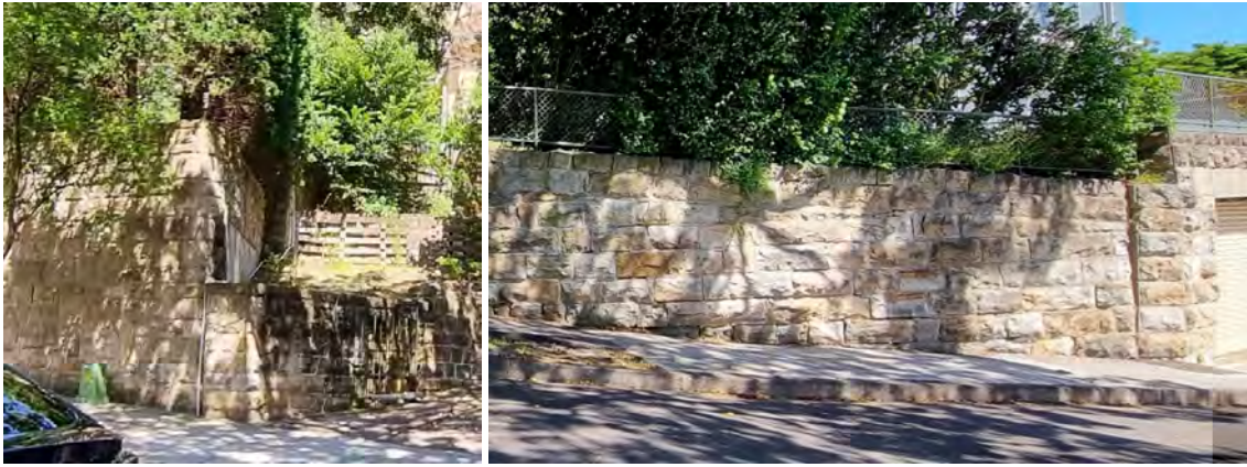
Figure 19 Sandstone block retaining walls
