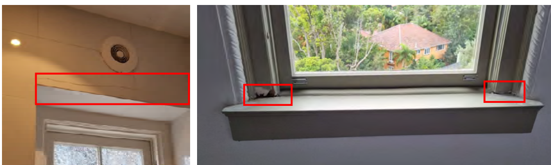
Figure 24 Tiles and timber window frame
