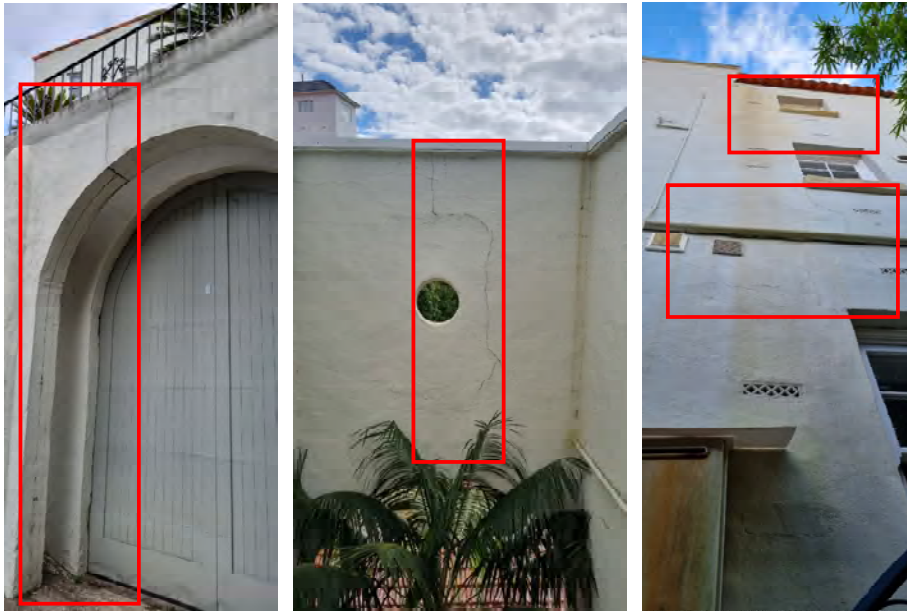
Figure 21 Exterior rendered brick walls
