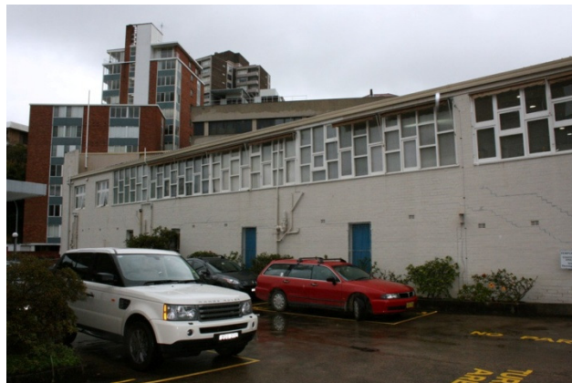
Figure 4 – The Thane Building as viewed from the adjoining property's visitor car parking area
