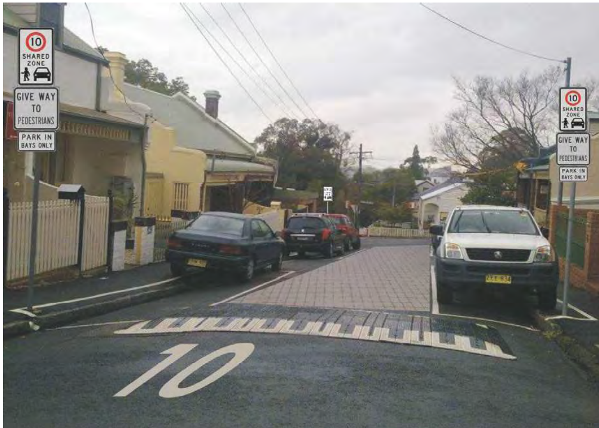
Figure 2. Photo and diagram of a Category 2 shared zone showing treatments, traffic calming, parking provision, and typical layout. 'Give Way' to Pedestrian' pavement marking is optional.
