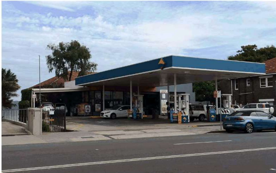
Figure 3: Existing petrol station at 638-646 New South Head Road
