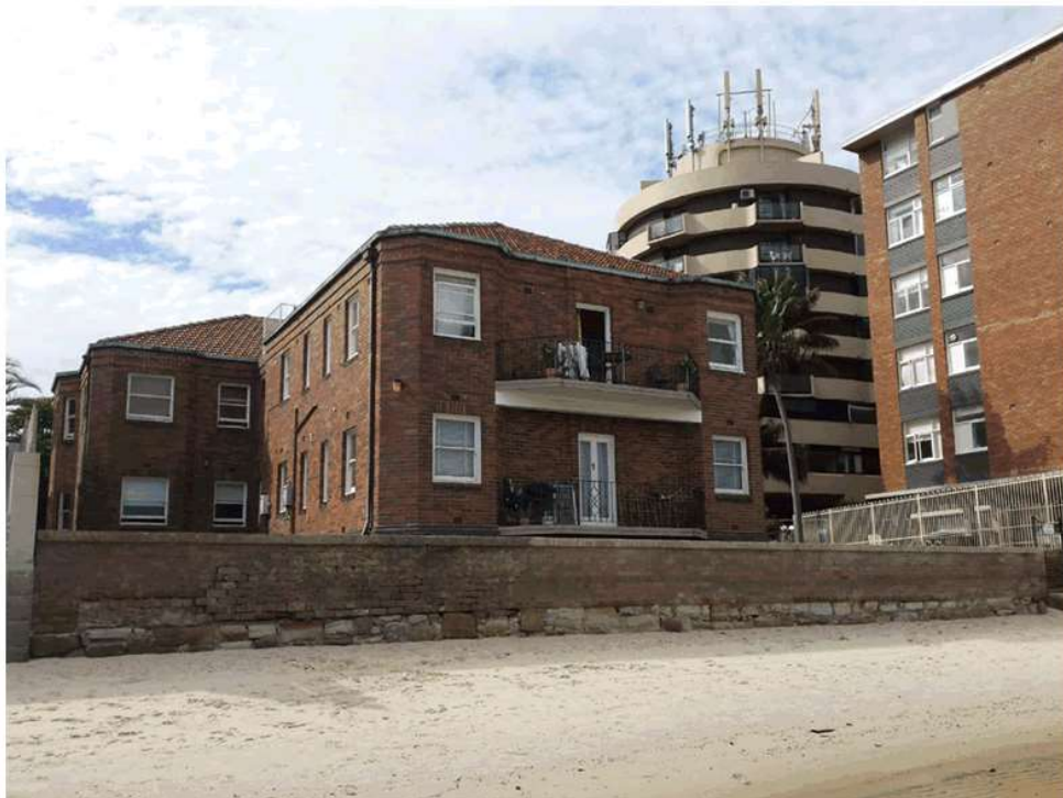
Figure 4: Existing residential flat building at 636 New South Head Road viewed from beach area at Rose Bay
