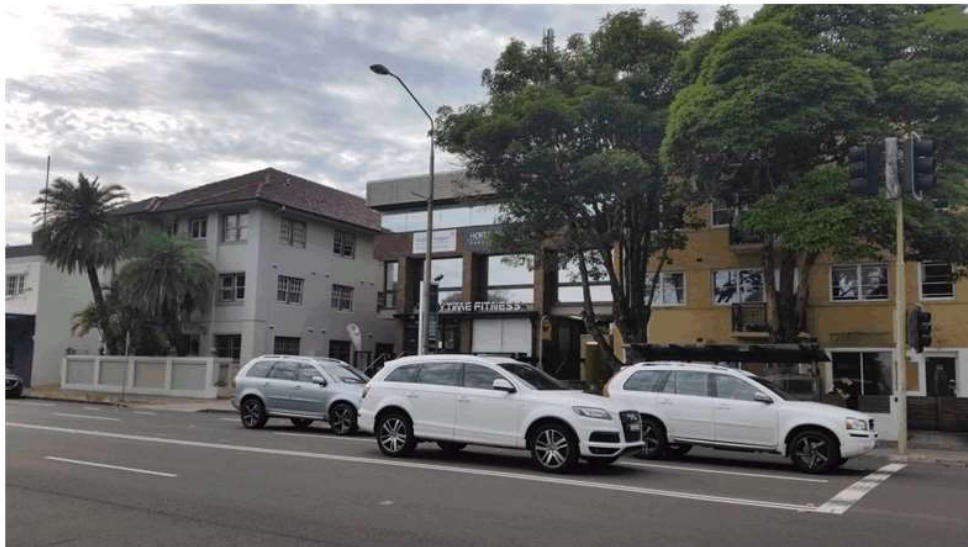
Figure 5: Existing development to the south of the site on New South Head Road, showing examples of typical nearby 2-3 storey mixed use and residential flat buildings (source: JBA)
