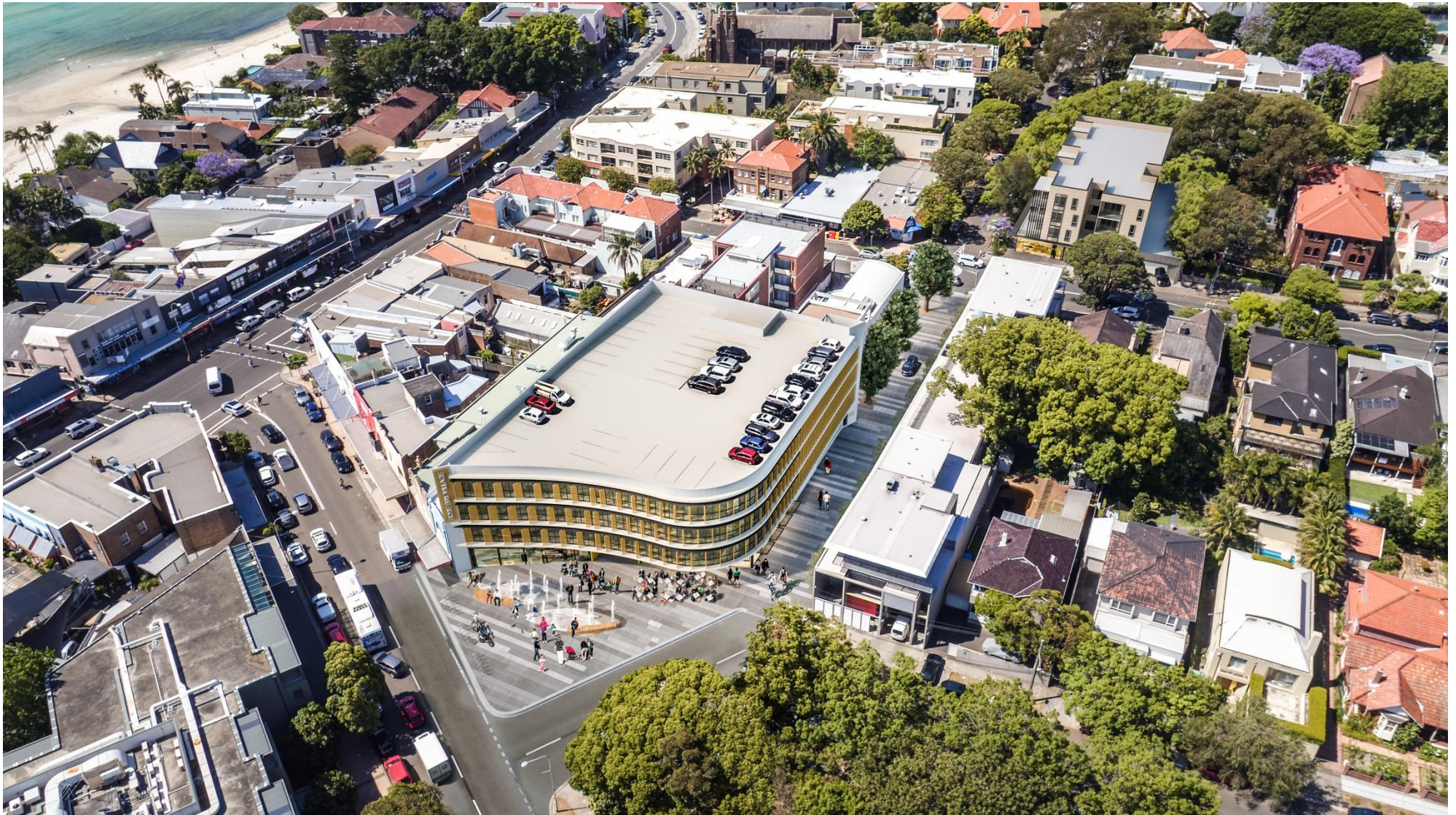
Image 6: Aerial photomontage of the concept for the Wilberforce Avenue Car Park and Ian Street Car Park sites (looking north-east)
