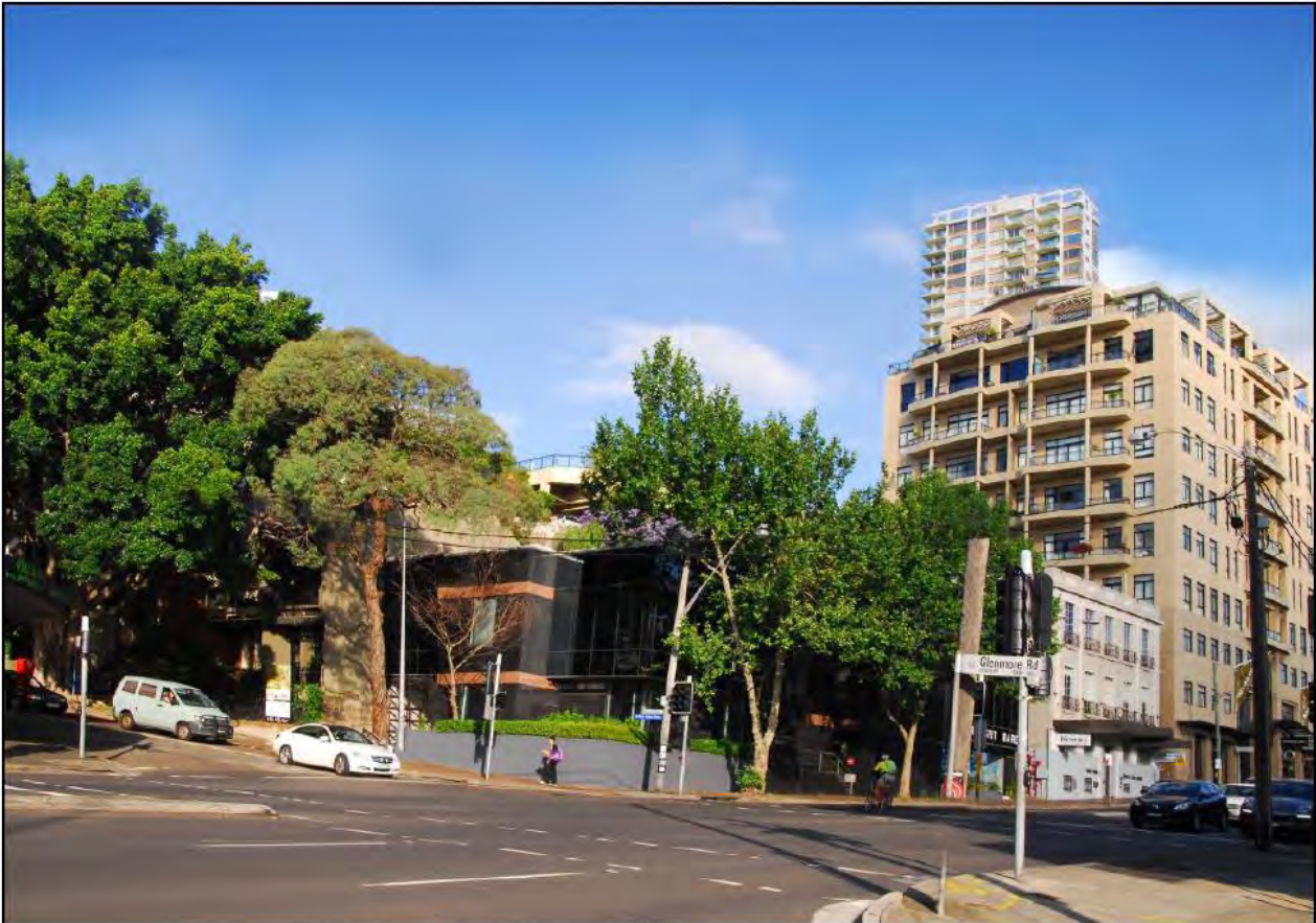
Figure 5: Existing perspective of the south-west corner (source PTI Architects)
