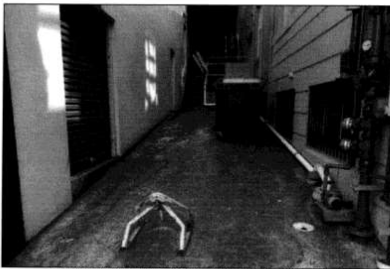
Photograph 1: The Right of Way Access from New South Head Road
