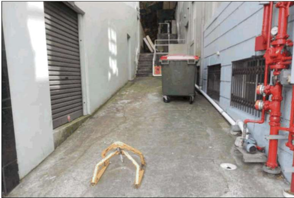
Photograph 1: The Right of Way Access from New South Head Road
