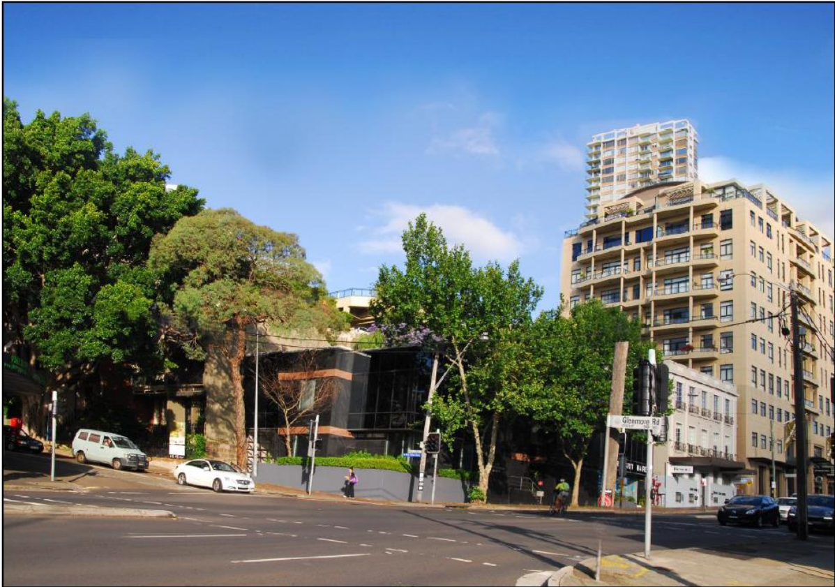
Figure 1: Existing perspective of the south-west corner (source PTI Architects)
