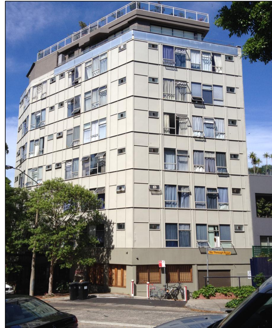
Photograph 6: 2B Mona Road, Darling Point
