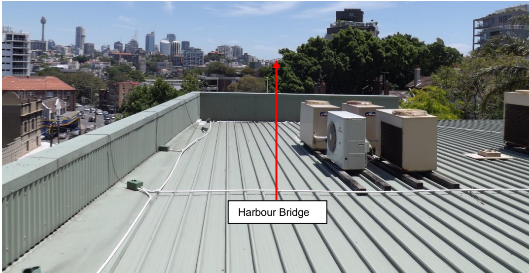
Photograph 1: Taken standing on the roof of No. 90 New South Head Road, in front of the far southern window on the western facade of No. 100. This photograph is taken approximately 1.8 metres below the sill height of the window of No. 100
