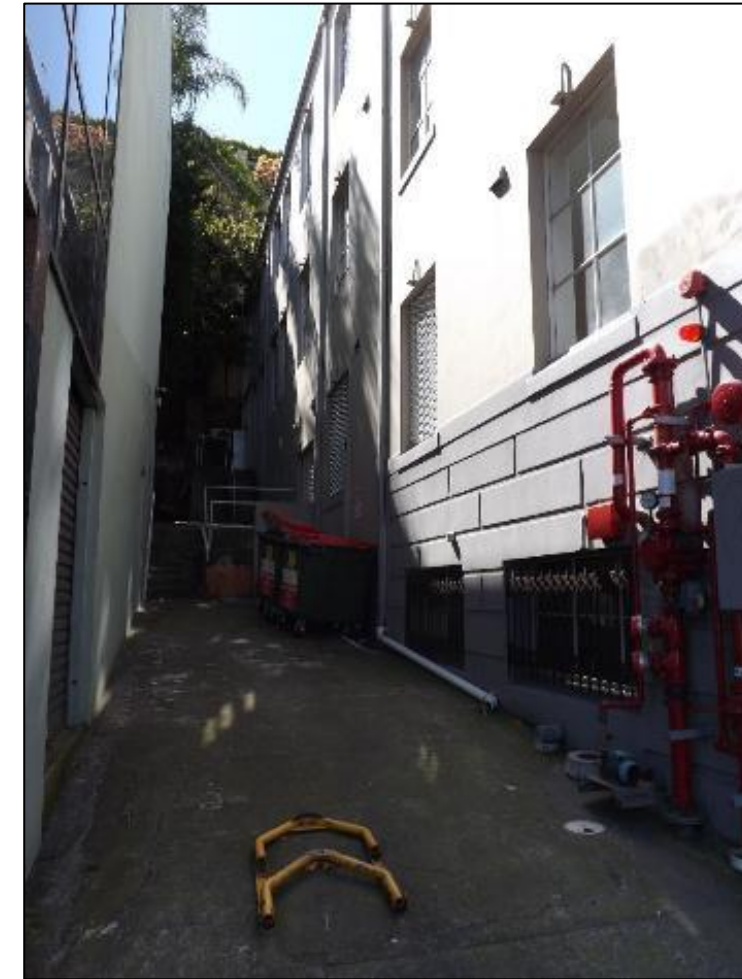
Photograph 4: Right of Way, 90 New South Head Road
