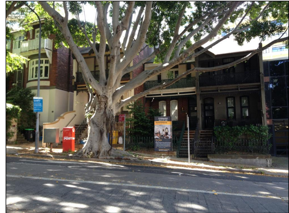
Photograph 9: Heritage Listed Terraces - 9-11, 15 & 17 Mona Road, Darling Point
