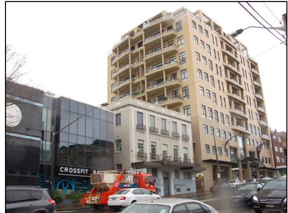
Figure 16. View from south-west along New South Head Road. (Source: Rappoport Pty Ltd, 19 August 2014)
