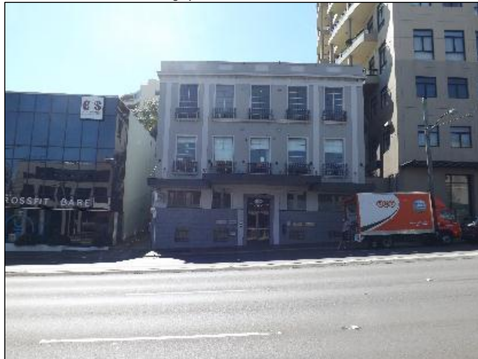
Photograph 3: 90 New South Head Road
