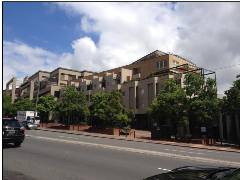
Photograph 8: 161 New South Head Road, Edgecliff
