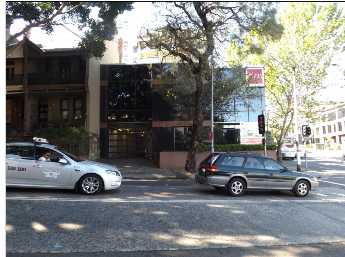
Photograph 10: Existing Interface with the adjoining Heritage Item at 9 Mona Road
