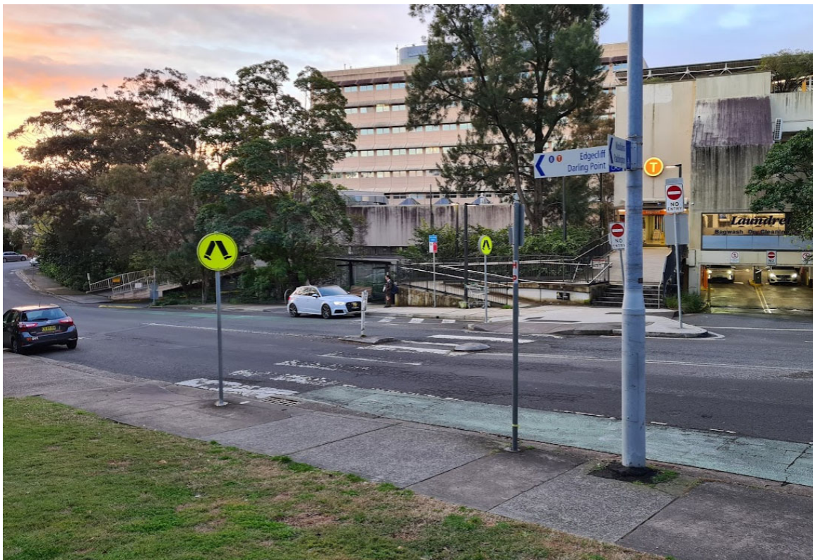
Figure 4 Edgecliff station entrance on New McLean Street
