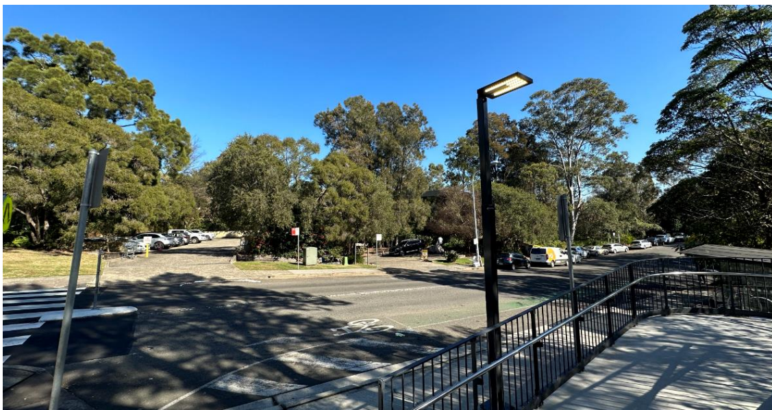
Figure 7 Existing elevated carpark deck of Nos. 8-10 New McLean Street, Edgcliff, as viewed from streetscape
