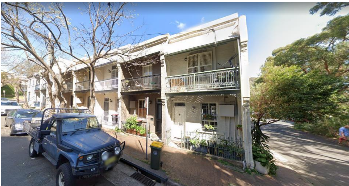
Figure 4.3: Heritage Terraces on Arthur Street. Source: Google Maps 2022
