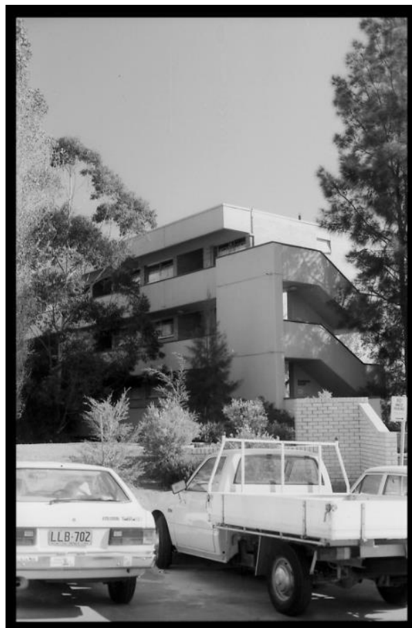
Figure 3.11: View of 8-10 New McLean Street from the carpark in 1982.
