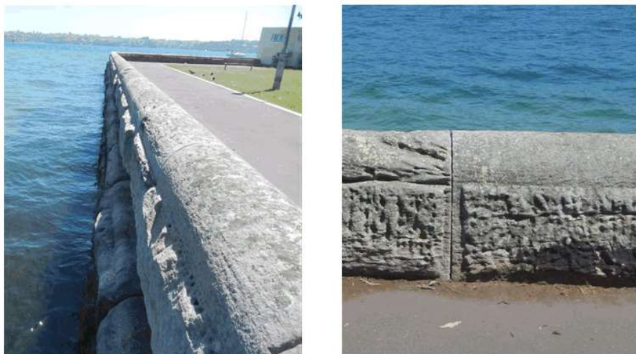
Figure 2. Photographs of the seawall
