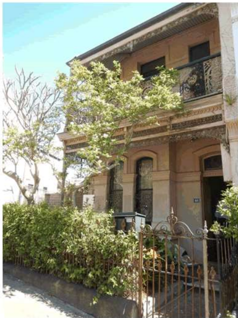
Figure 2. Front façade of 48 Duxford Street, Paddington
