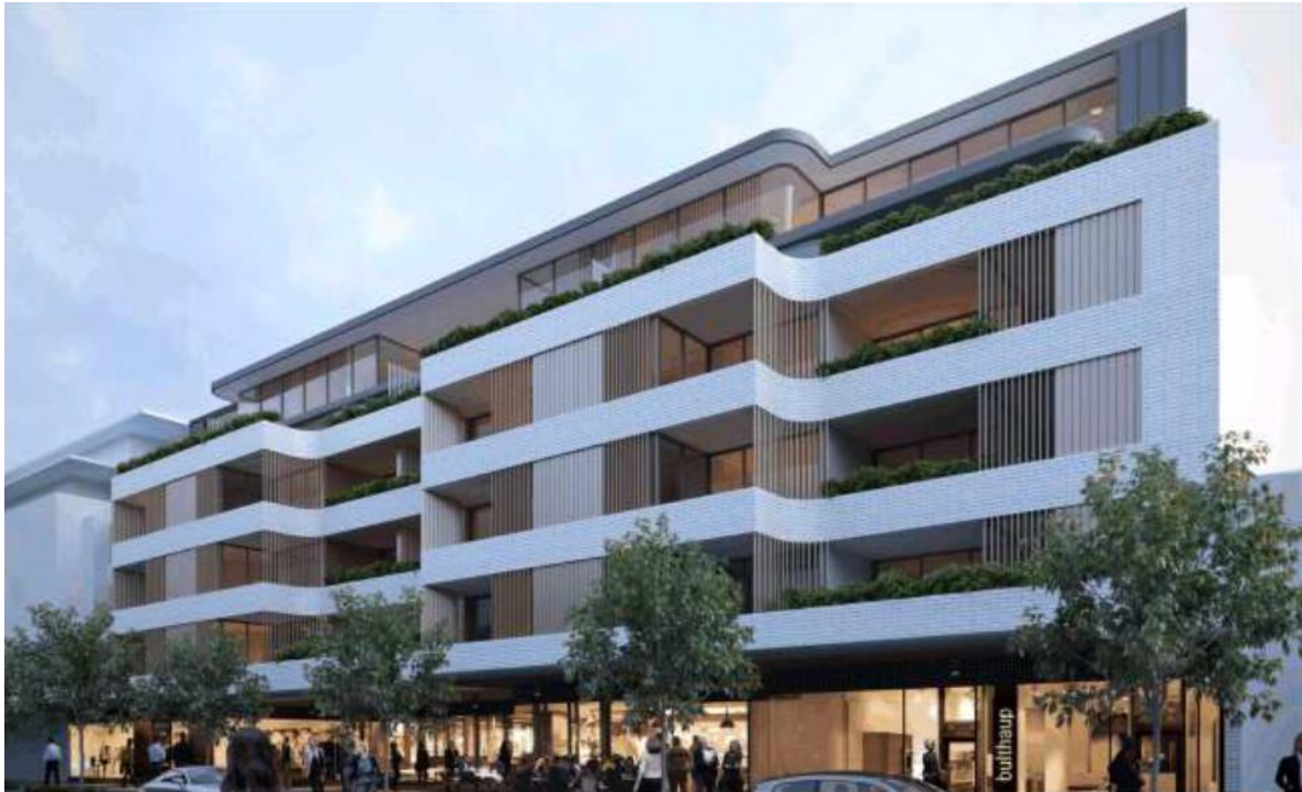
Figure 8 – Hunters Lodge (16-18 Cross Street) Source: Bates Smart
