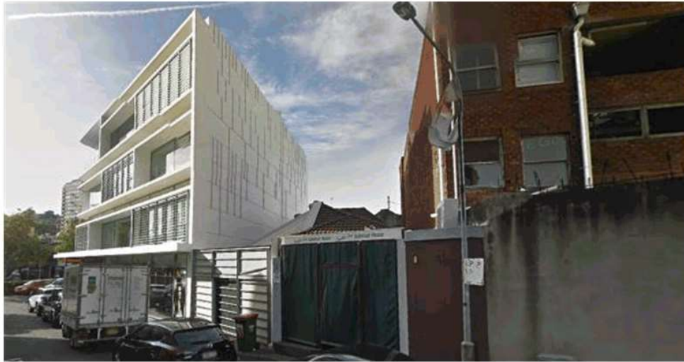
Figure 4 – View of site from Goldman Lane looking southeast Source: Google
