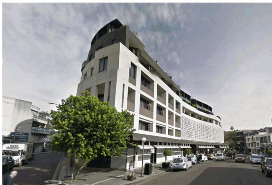
Figure 7 – The Stamford Cosmopolitan Centre (2-22 Knox Street) Source: Google maps
