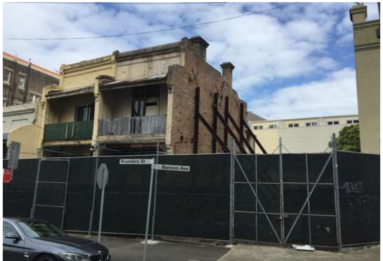
Figure 4: Existing dilapidated double storey terraces at 196-200 Boundary Street (source SJB)
