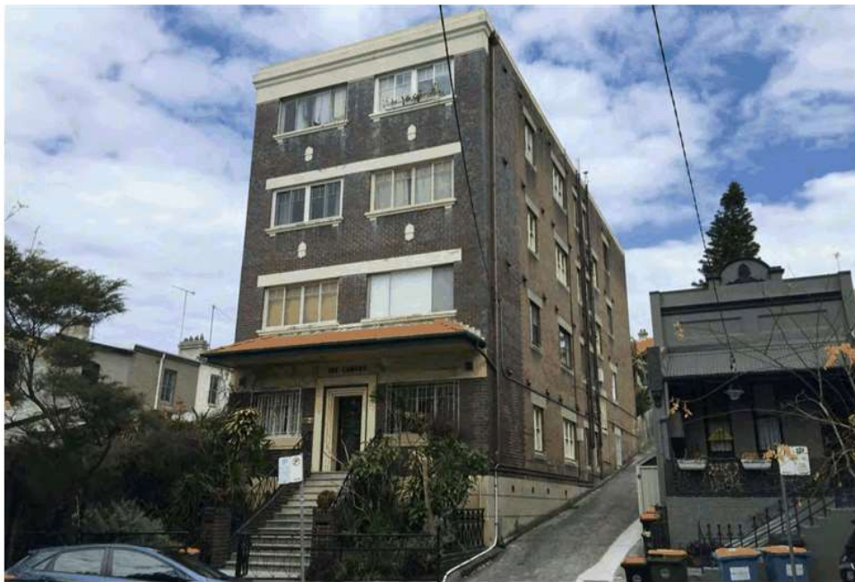
Figure 6: Residential flat building at 186 Boundary Street.
