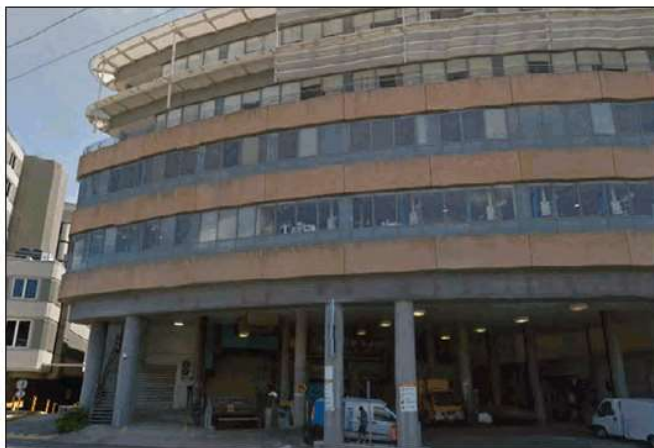
St. Vincent's Hospital along Boundary Street
