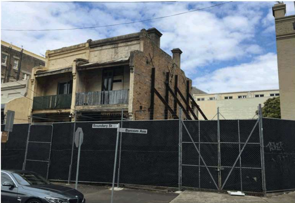
Figure 4: North eastern elevation of terrace dwellings at 196 – 200 Boundary Street
