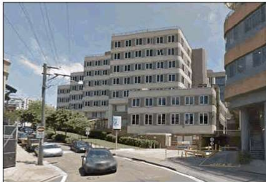
St. Vincent's Hospital along Boundary Street
