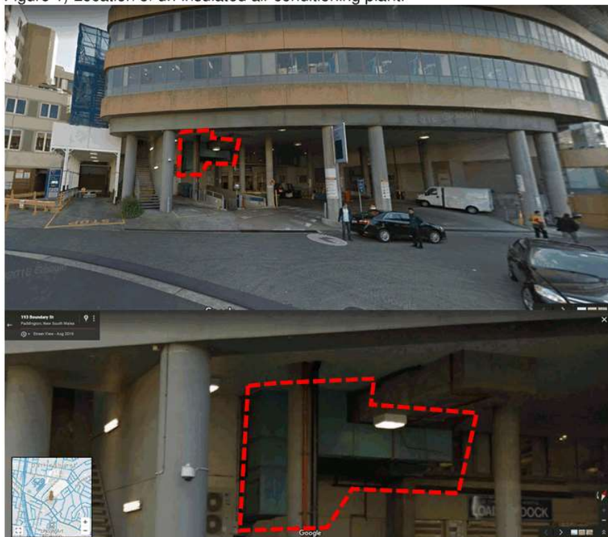
Figure 1) Location of un-insulated air conditioning plant.
