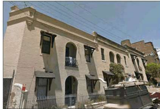
Adjoining residential buildings along Boundary St.
