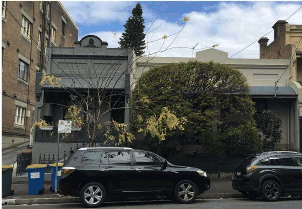
Figure 3: Existing single storey terraces at 190-194 Boundary Street (source SJB)
