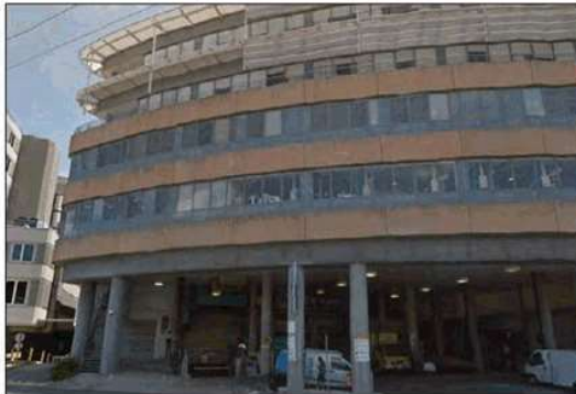
St. Vincent's Hospital along Boundary Street
