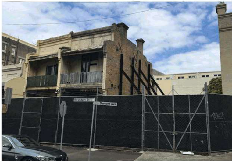
Figure 4: North eastern elevation of terraco dwellings at 196 – 200 Boundary Street
