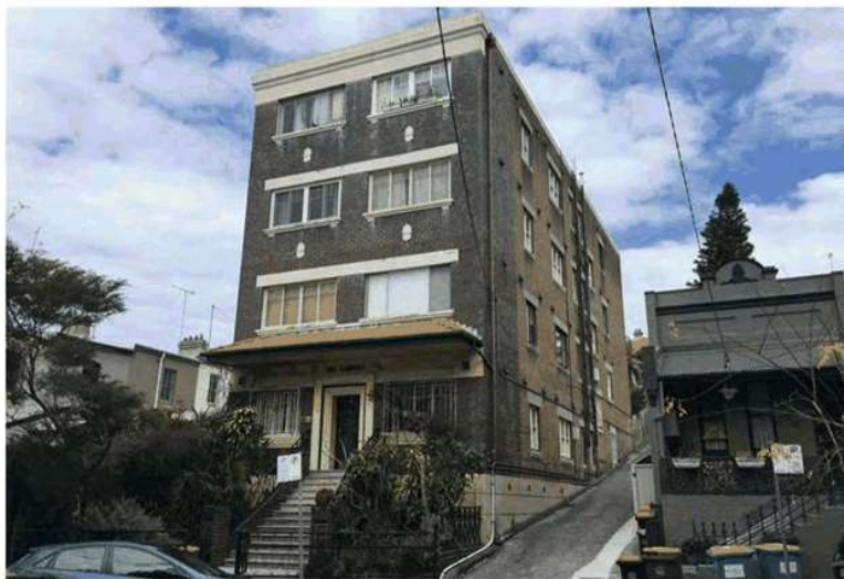
Figure 6: Residential flat building at 186 Boundary Street
