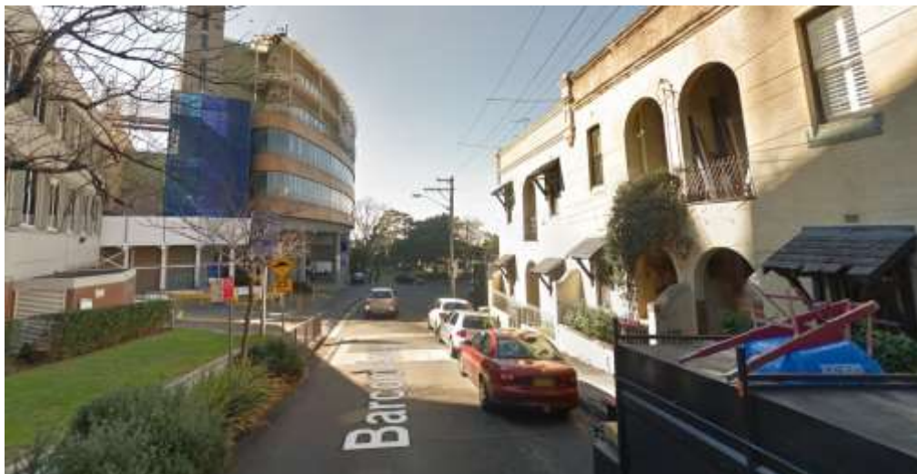
Figure 6: Context and street frontage for 278-282 Barcom Ave (Source: Google Street View)
