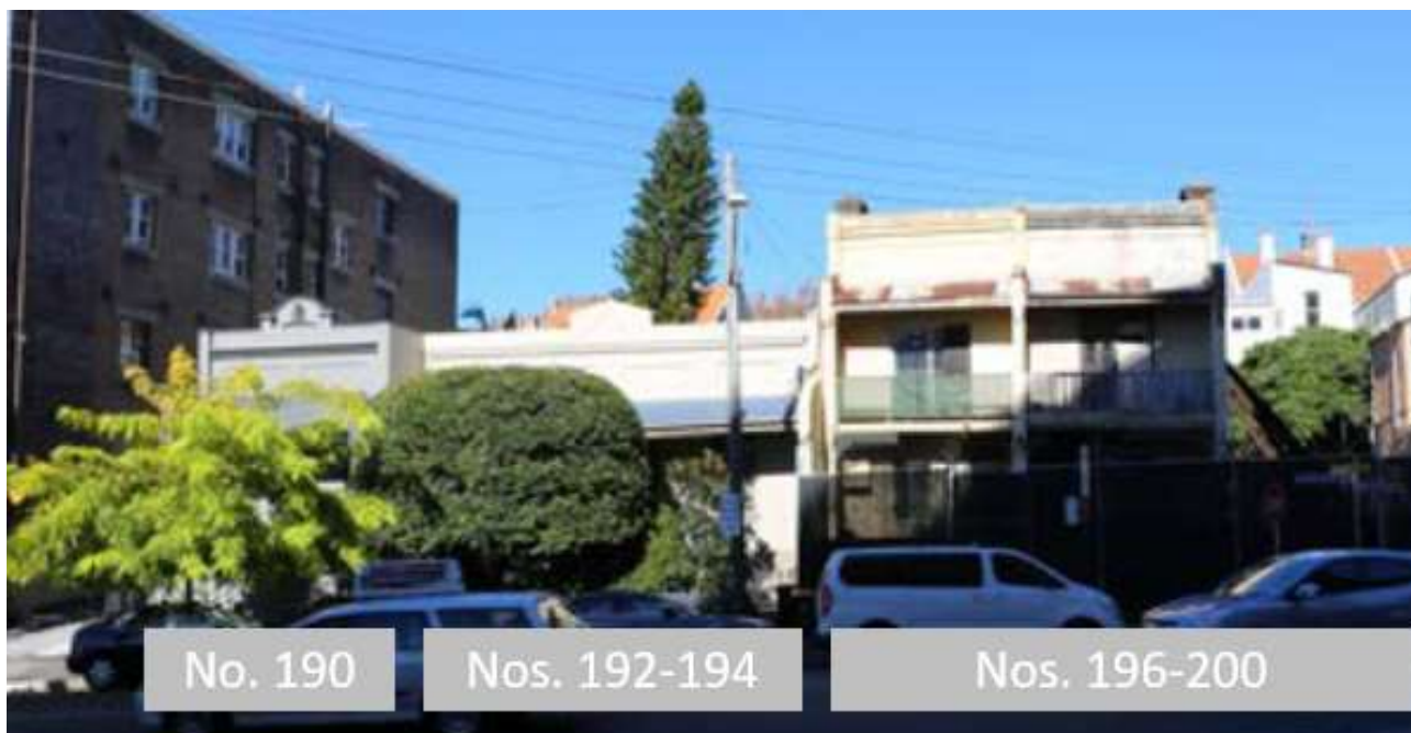
Figure 2: 190-194 Boundary St and 196-200 Boundary St (source SJB)
