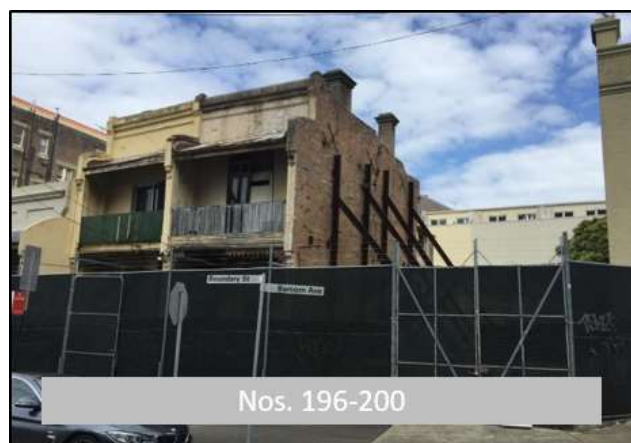
Figure 4: Existing double storey terraces at 196-200 Boundary St (source SJB)
