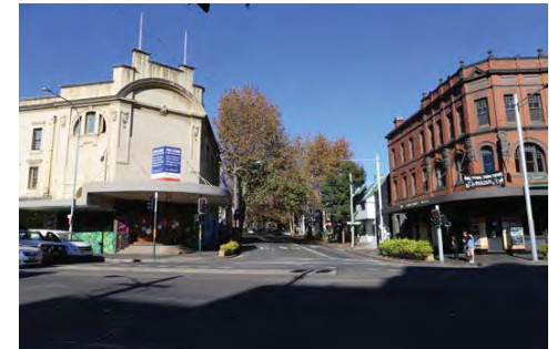
Condition of Barcom Avenue, Oxford Street and South Dowling Street junction
