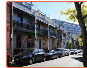
Terraces along West Street
