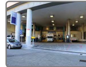
St Vincent's Hospital Loading Bay / BOH
