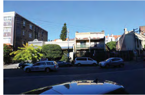
Northern facade of subject site along Boundary Street
