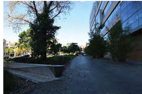
View of Barcom Avenue Park and St Vincent's Hospital from Ice Street
